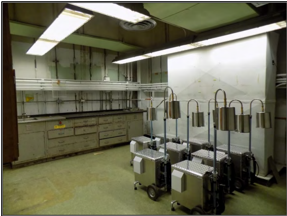
Figure A-28. Current photograph showing the Reactor Maintenance Plant and Equipment Division Office in the southeast corner of the south wing on the second floor of Building 3042, facing southeast.
