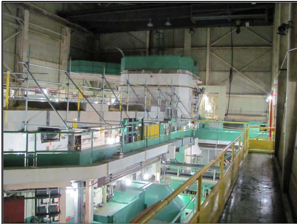
Figure A-14. Current photograph showing the high bay dominated by the ORR structure, facing southwest. In the center background the hot cell area occupies the west end of the reactor structure.
