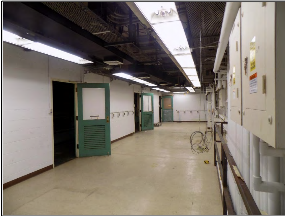
Figure A-29. Current photograph showing the Control Room for in-pile experiments located on the second floor of the north wing of Building 3042, facing west.
