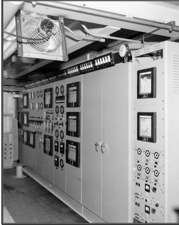
Figure A-49. Archival photograph showing the GCR-ORR Loop No. 1 control panel located in the Irradiation Engineering Room in the north wing of the basement in Building 3042, circa 1959 (ORNL Photo 48279).
