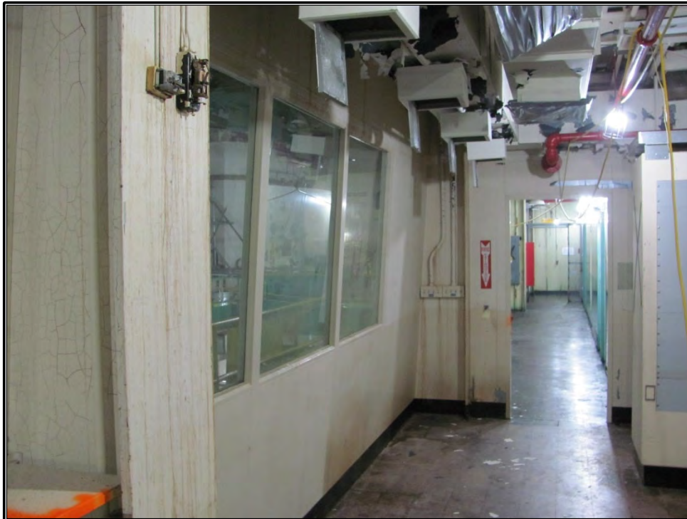
Figure A-33. Current photograph showing the viewing windows located in the third floor Control Room and a portion of the third floor north corridor in the north wing of Building 3042, facing west.
