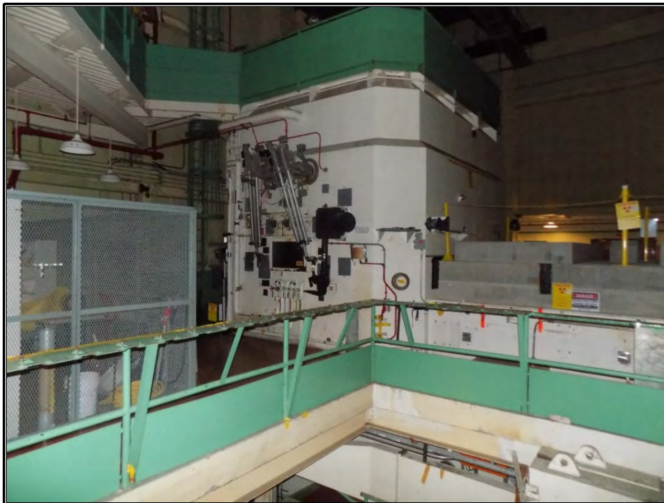
Figure A-34. Current photograph showing the hot cell area located on the west end of the ORR structure at the third-level of Building 3042, facing northwest.
