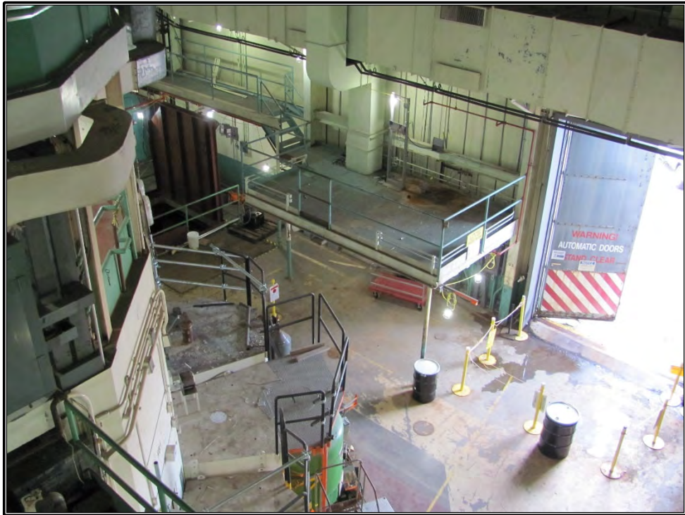
Figure A-15. Current photograph showing the east portion of the high bay in Building 3042, including the second-level platform on the east wall, as seen from the third floor south corridor, facing northeast.
