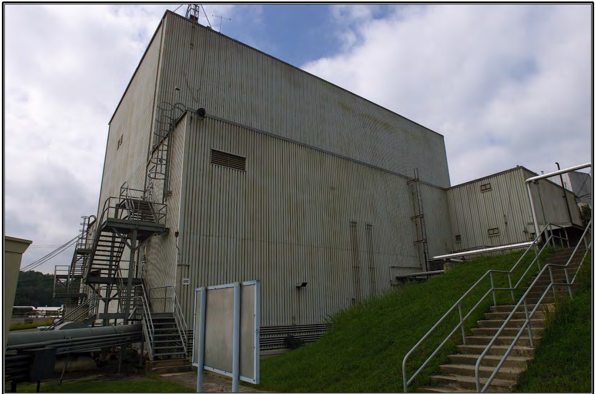
Figure A-7. Circa 2003 photograph showing the north and east elevations of Building 3042, facing southwest.
