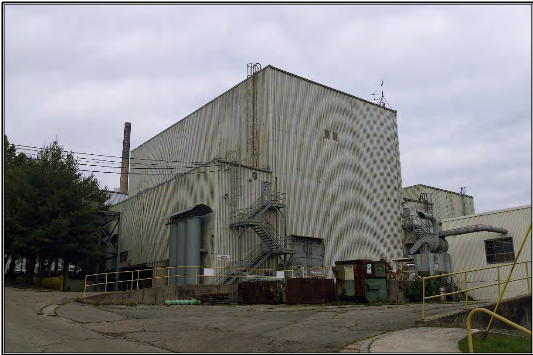
Figure A-1. Circa 2003 photograph showing the east and south elevations of Building 3042, facing northwest.
