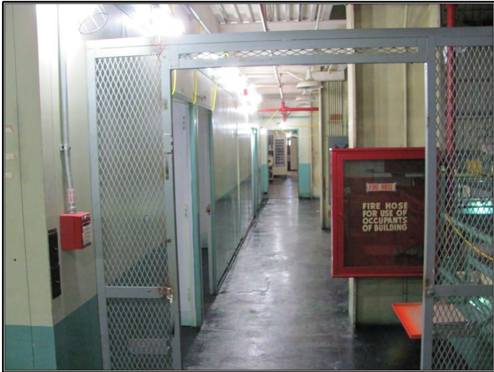
Figure A-31. Current photograph showing the west end of the third floor north corridor in Building 3042, facing east.
