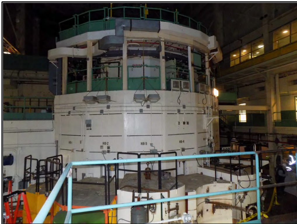
Figure A-12. Current photograph showing the east end of the ORR structure dominating the high bay of Building 3042 as seen from the second-level platform on the east wall, facing west.
