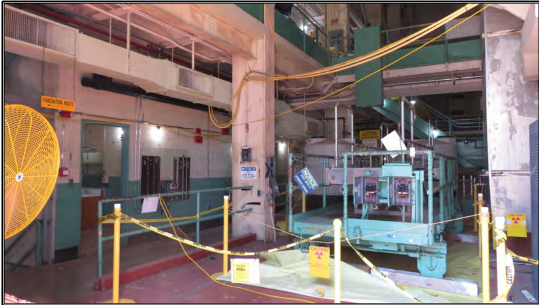
Figure 120. Current photograph of second floor of Building 3042, looking northeast from the service entry on the west side of the building. In the foreground is the truck alley. At left is a restroom. At upper right is a suspended walkway connecting the third floor of the north wing to the reactor structure.
