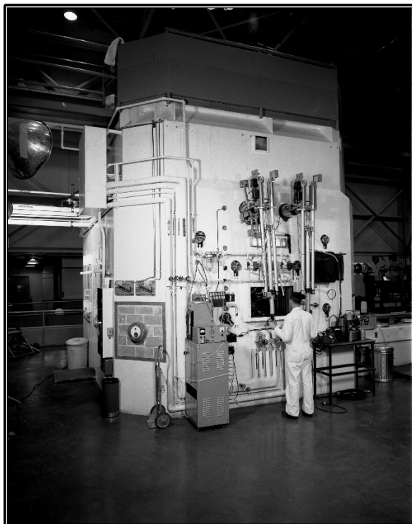
Figure 178. Archival photograph showing the hot cell area at the west end of the reactor structure in Building 3042 (ORNL Photo 48951).
