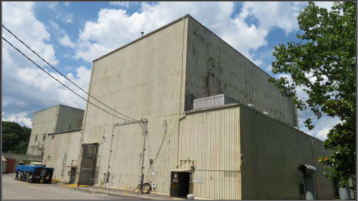
Figure 52. Current photograph of west elevation of Building 3042, including the west elevation of the circa 1957 Change House addition at left, facing northeast.
