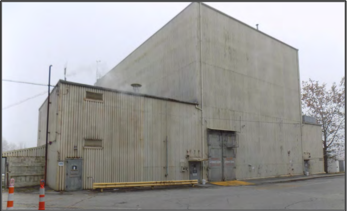
Figure 53. Current photograph of west elevation of Building 3042, facing southeast.
