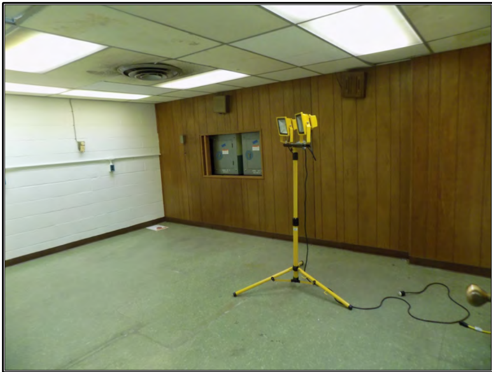
Figure 117. Current photograph showing Room 208 on the second floor of the south wing in Building 3042, facing southeast.
