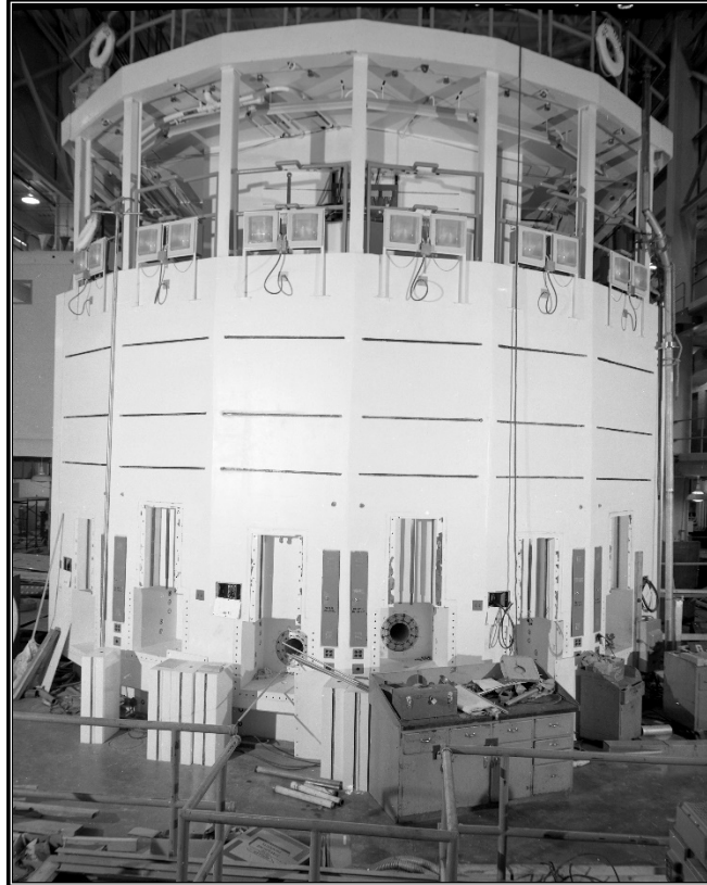
Figure 190. Archival photograph showing most of the HB facilities piercing the face of the reactor structure in Building 3042, circa 1957 (ORNL Photo 42186).
