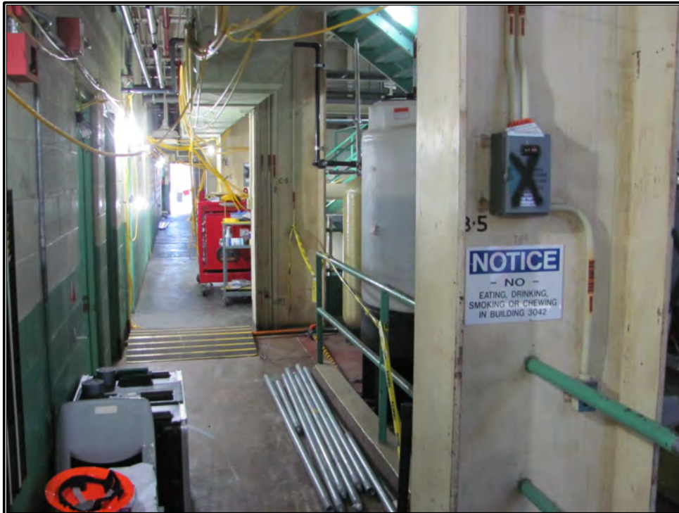
Figure 106. Current photograph showing the north corridor on the second floor of Building 3042, facing east. The stairwell leading to the reactor structure is in the background at right.
