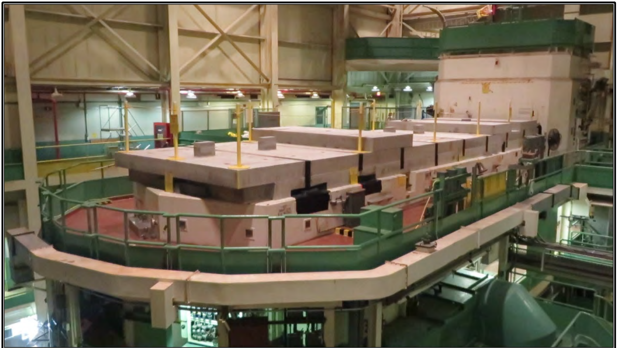
Figure 39. Circa 2015 photograph showing the reactor pool capped with concrete shielding panels, facing southwest (UCOR 2016:22).
