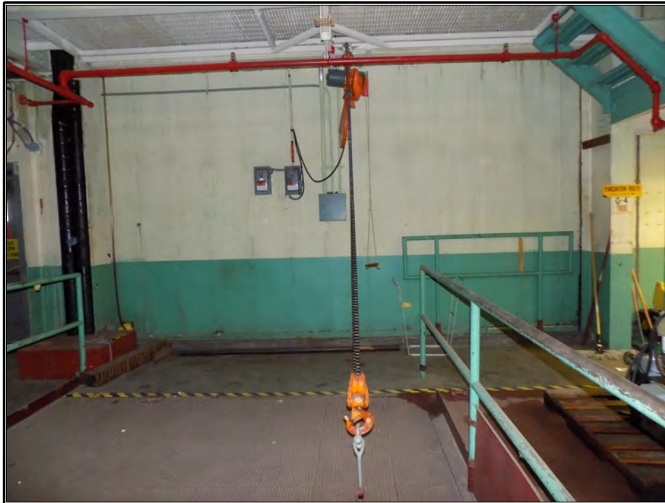
Figure 94. Current photograph showing the hatch located in the northeast corner of the high-bay on the first floor of Building 3042, facing east.
