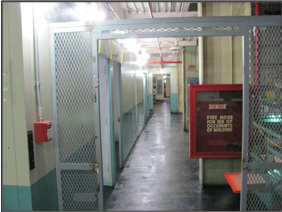
Figure 126. Current photograph showing the metal grate wall situated at the west end of the third-floor north corridor, facing east.
