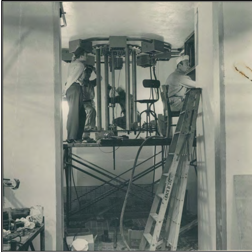
Figure 62. Archival photograph showing the sub-pile room in the basement of Building 3042, circa 1957 (ORNL Photo 57-1477).
