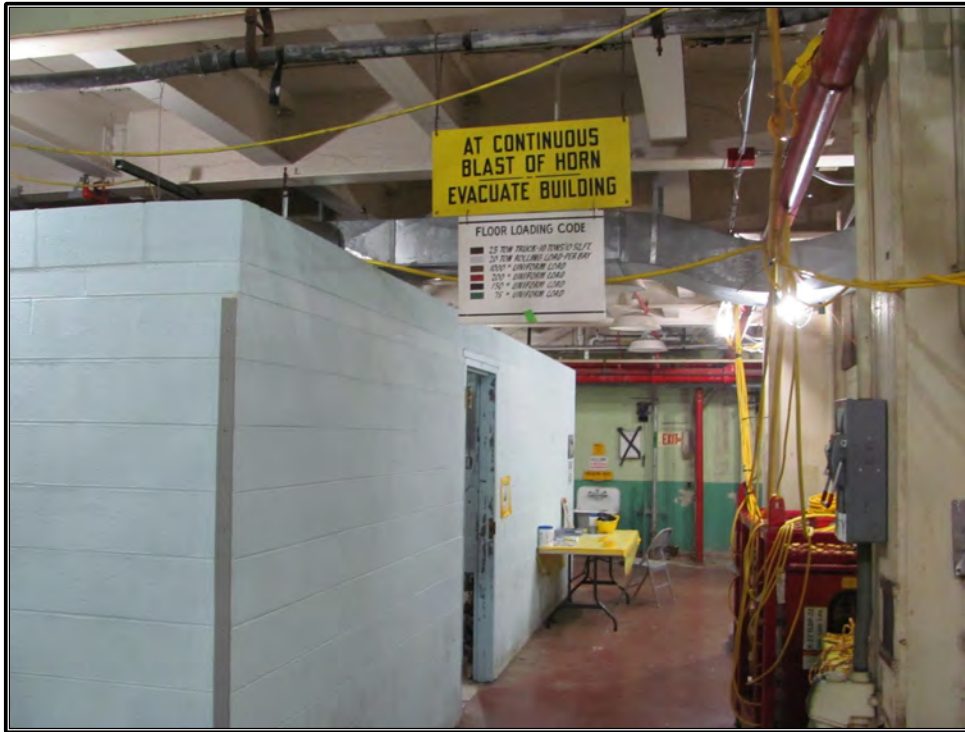
Figure 91. Current photograph showing the north first floor corridor, facing west. At left is the Electrical Shop located on the northwest corner of the reactor structure.
