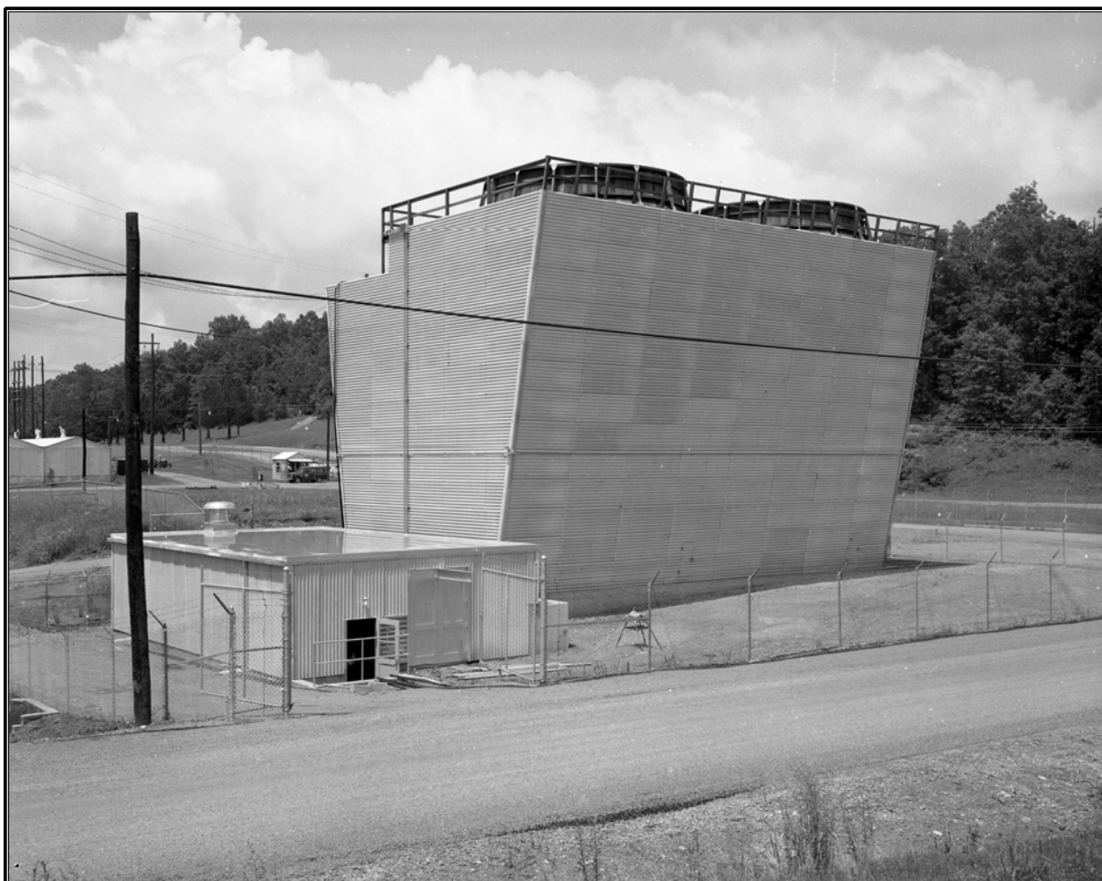
Figure 36. Archival photograph of a new cooling tower and pump house for the ORR, which would accommodate an increase in the reactor's power level from 20 Mw to 30 Mw, July 13, 1960 (ORNL Photo 50640).
