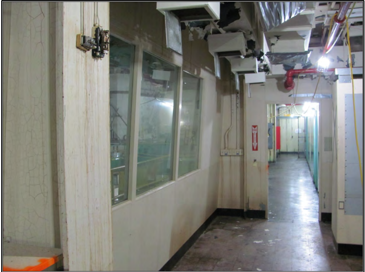
Figure 128. Current photograph showing the west portion of the south wall in Room 309, the Control Room, facing west toward the third-floor north corridor.
