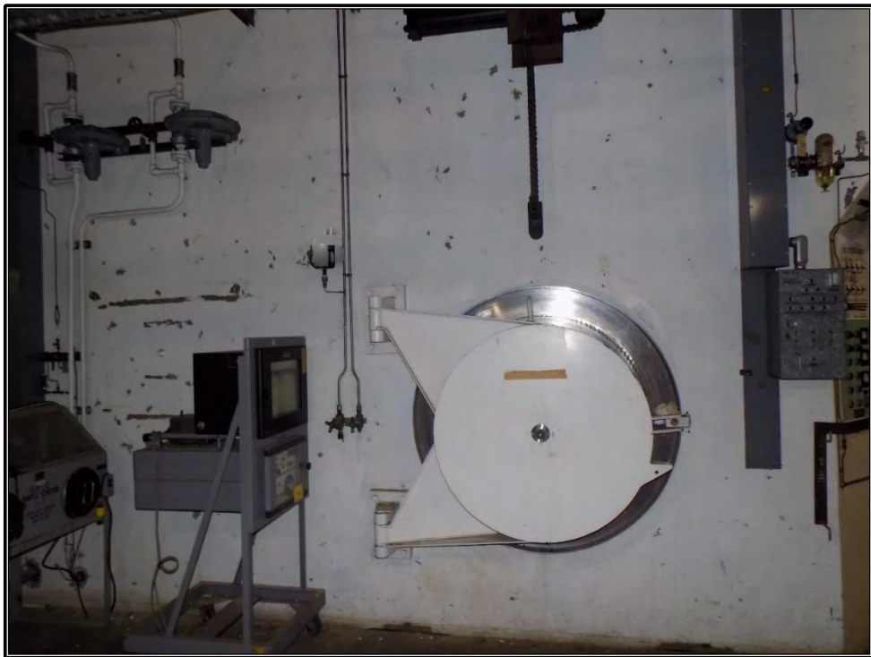
Figure 146. Current photograph showing one two Engineering Test Facilities on the reactor structure.
