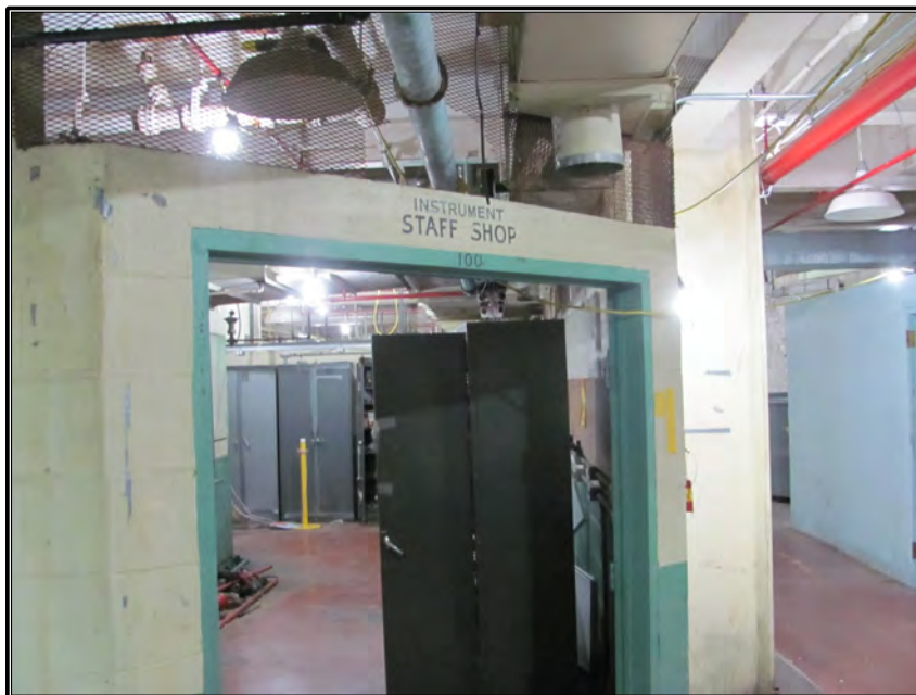
Figure 86. Current photograph showing the entrance to the Instrument Staff Shop or Room 100, previously the General Staff Shop, facing east.
