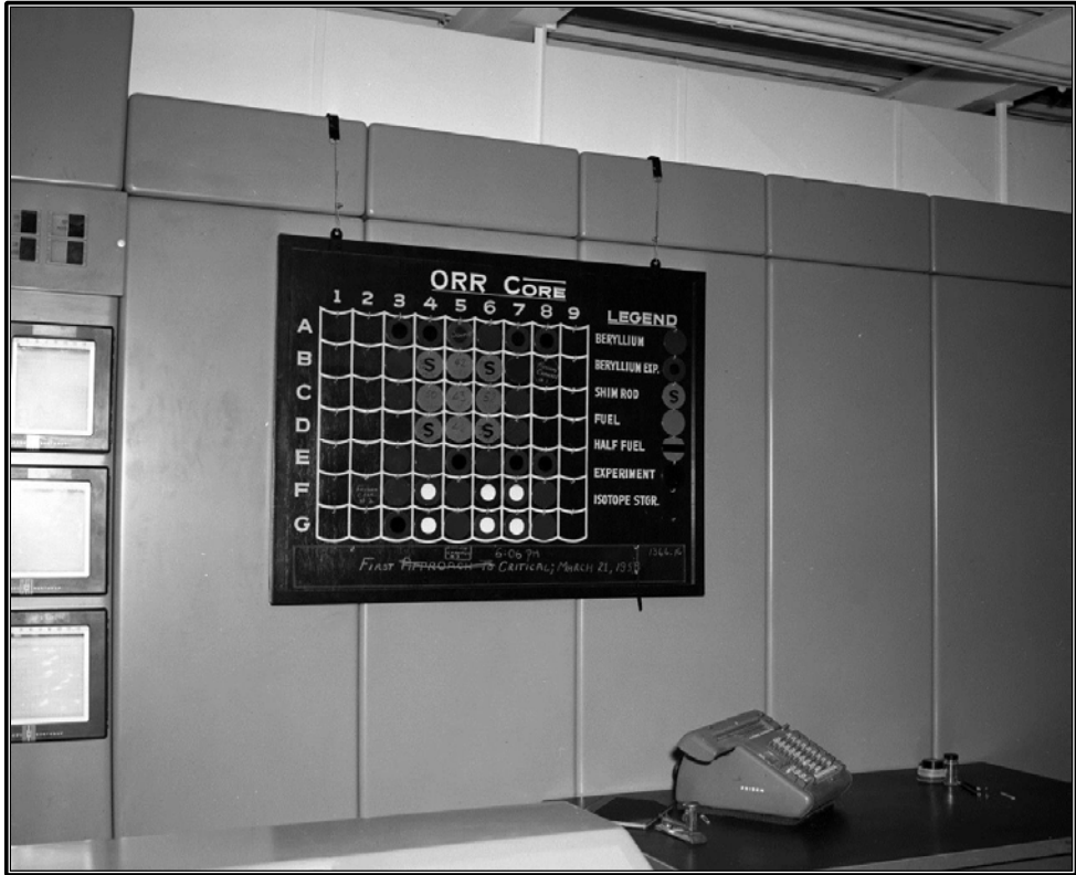
Figure 184. Archival photograph showing the ORR Core configuration board in the Control Room of Building 3042 on the day the reactor went critical, March 21, 1958 (ORNL Photo 3210).
