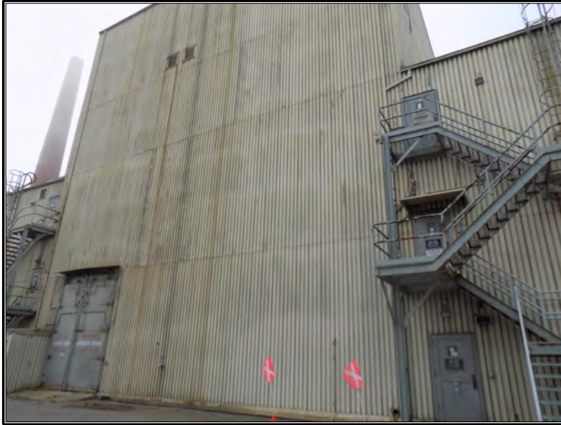
Figure 41. Current photograph of east elevation of Building 3042, facing southwest.
