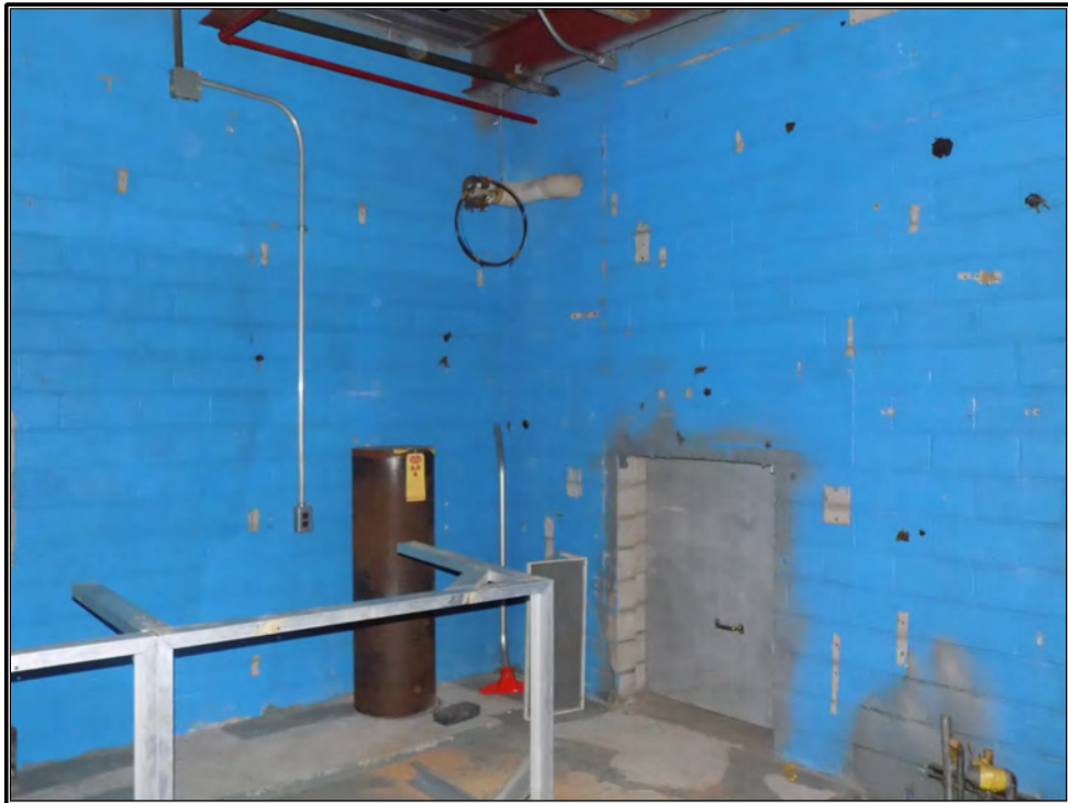
Figure 71. Current photograph showing the Reactor Chemistry Room facing northwest.
