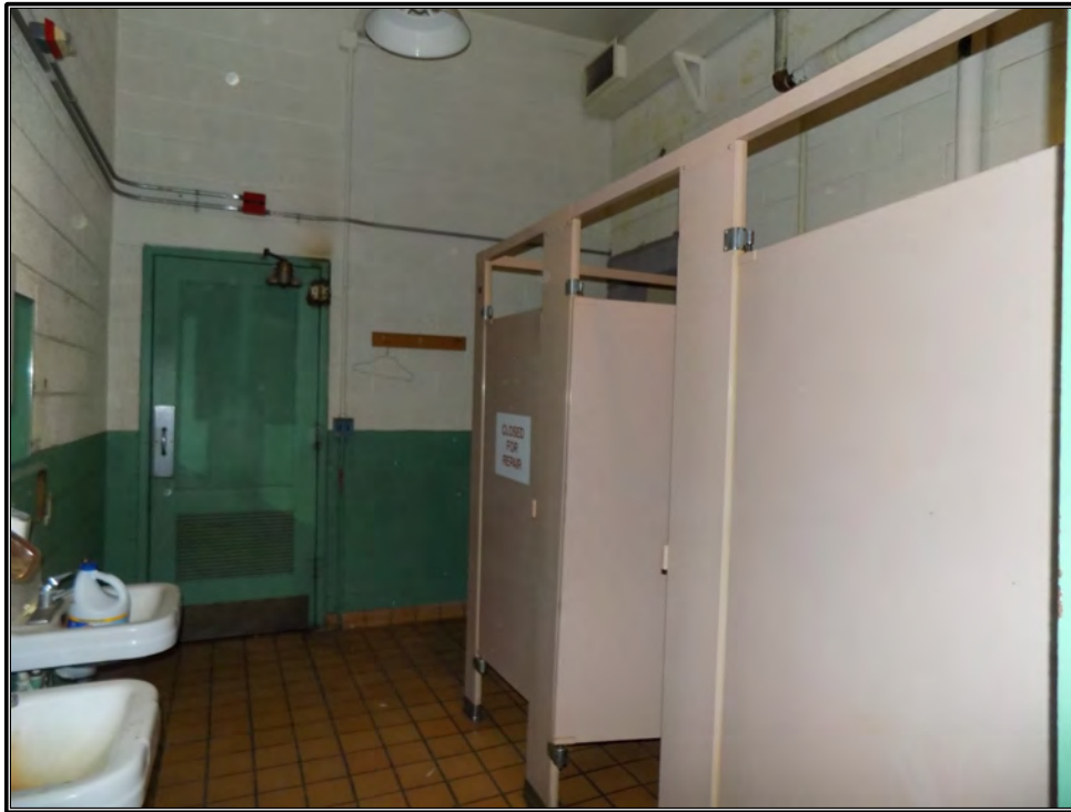
Figure 108. Current photograph showing the men's restroom in the northwest corner of the second floor of Building 3042, facing south.
