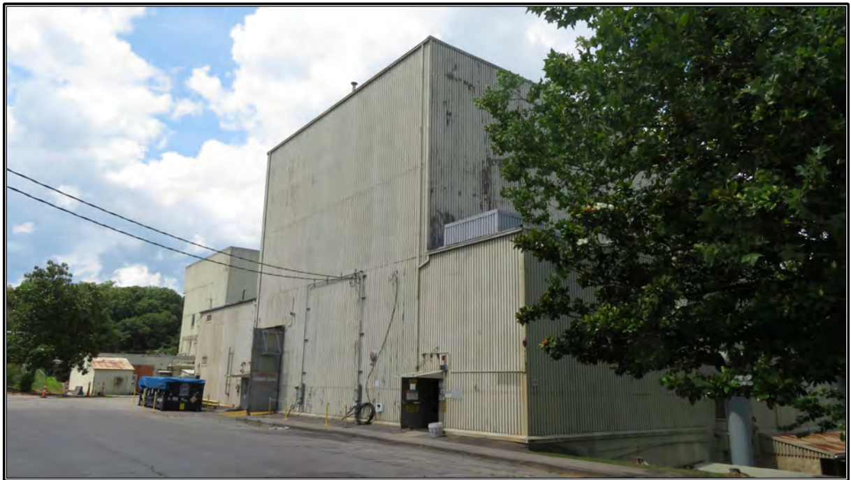
Figure 11. Current photograph of the exterior of Building 3042, facing northeast.
