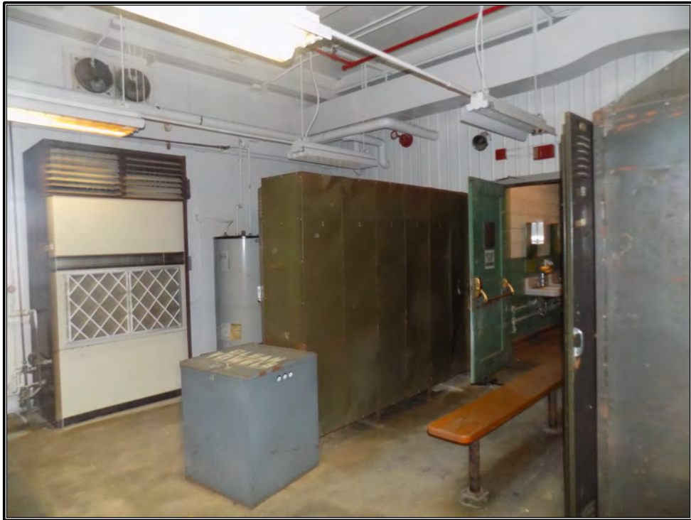
Figure 123. Current photograph of lockers in the men's change room on the second floor of a northwest addition made to Building 3042 in 1957; in the background is the doorway into the men's restroom.
