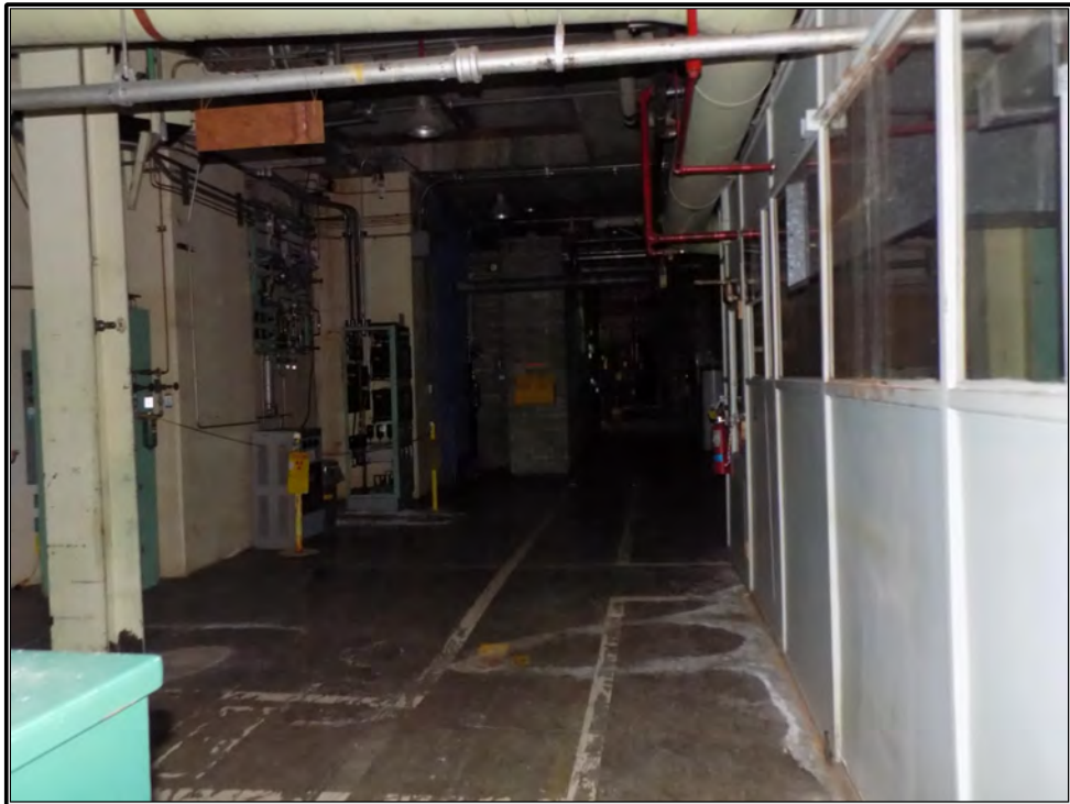
Figure 73. Current photograph showing the north basement corridor in Building 3042, facing west.
