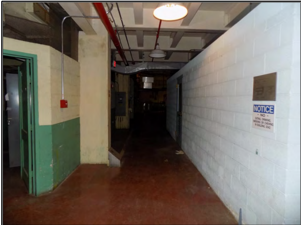
Figure 90. Current photograph showing the north first floor corridor, facing east. At left is the Instrument Staff Shop; at right is the Electrical Shop located on the northwest corner of the reactor structure.
