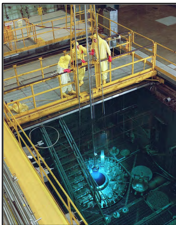
Figure 179. Archival photograph of the HFIR after completion, circa 1965. The HFIR was designed to provide a higher steady-state neutron flux than the ORR. Still in operation at the time of this writing, the HFIR is used to produce super heavy elements and for neutron science and material research (Rumsey 2018).
