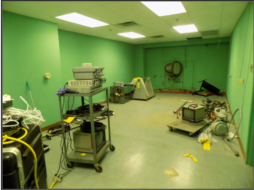
Figure 89. Current photograph of the enclosed space in the northwest corner of the first floor of Building 3042, previously designated the HB-6 Room, facing northeast. At center, time-of-flight equipment pierces the east wall and extends beyond the east elevation of Building 3042, connecting to Building 3107 to the northeast.
