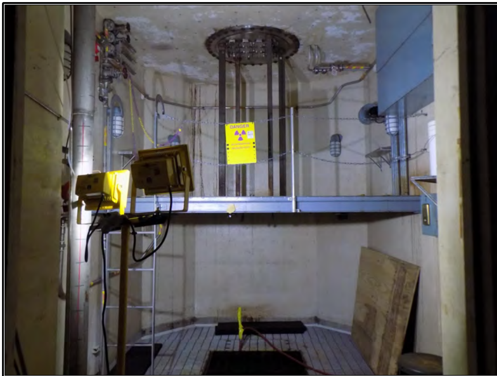
Figure 63. Current photograph showing the sub-pile room in the basement of Building 3042.
