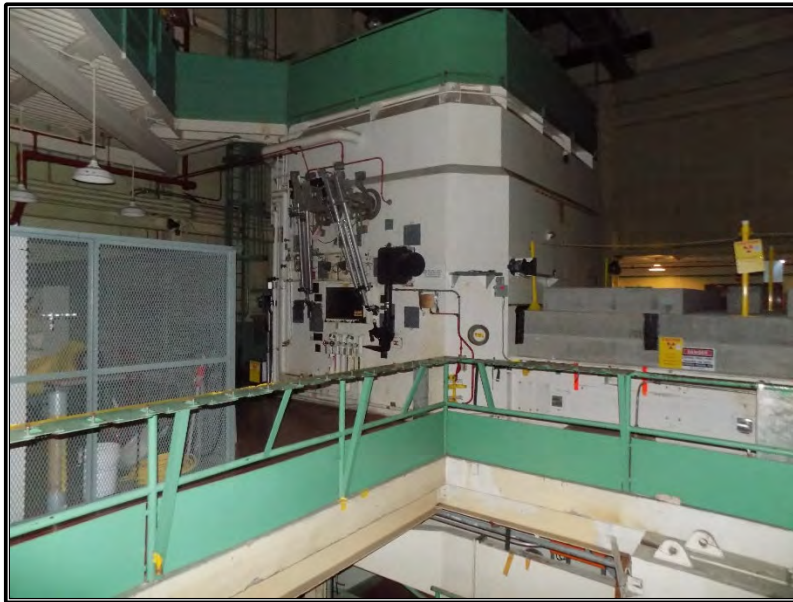
Figure 134. Current photograph showing the hot cell structure located at the west end of the reactor structure in Building 3042, facing northwest. The concrete shielding blocks are at right; the semi-hot storage platform is at left; and the crane access ladder and platform are at top left. The hot cell face shown is of the south hot cell.
