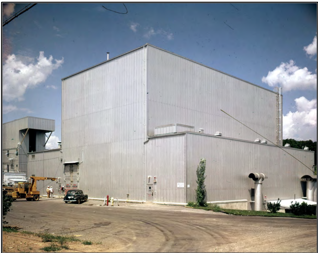
Figure 30. Archival photograph showing the west and south elevations of Building 3042, circa 1960. At bottom right, the shed-roof addition constructed at an unknown date protrudes from the south elevation (ORNL Photo 51411).
