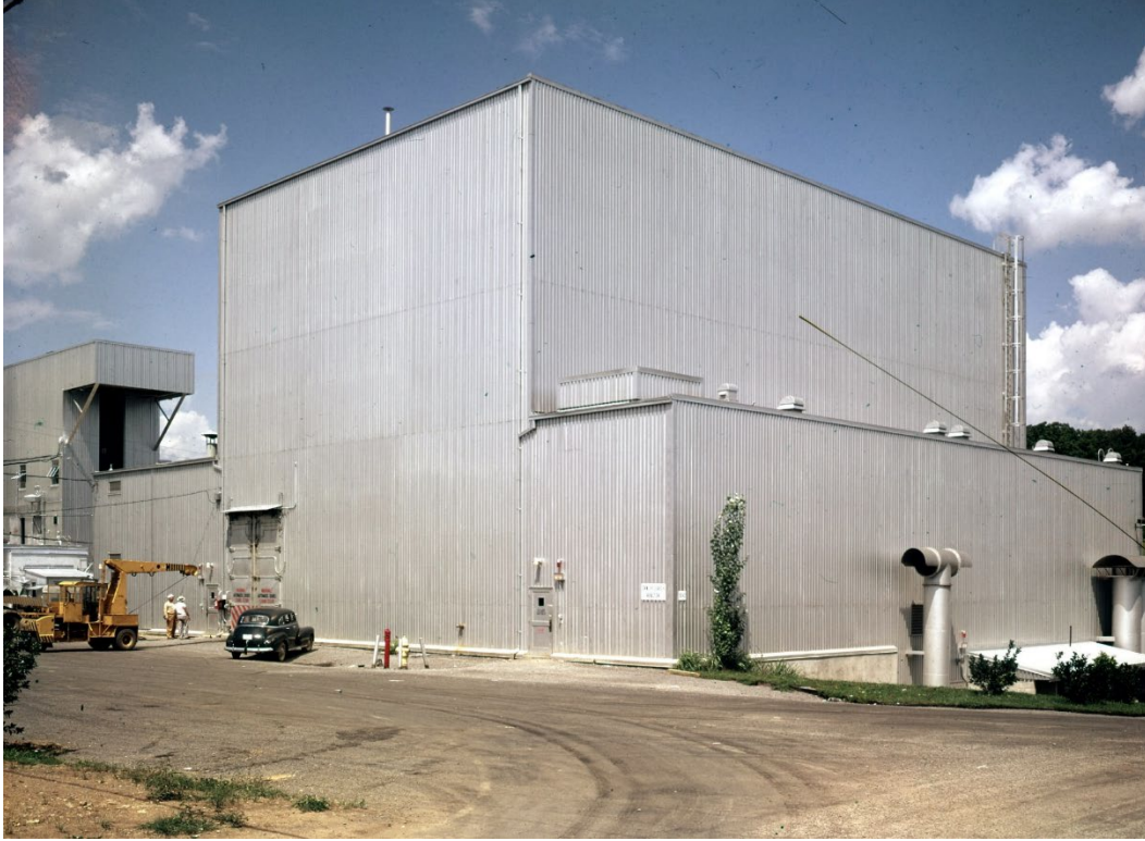
Fig. 2. The west and south elevations of Bldg. 3042, circa 1960.
