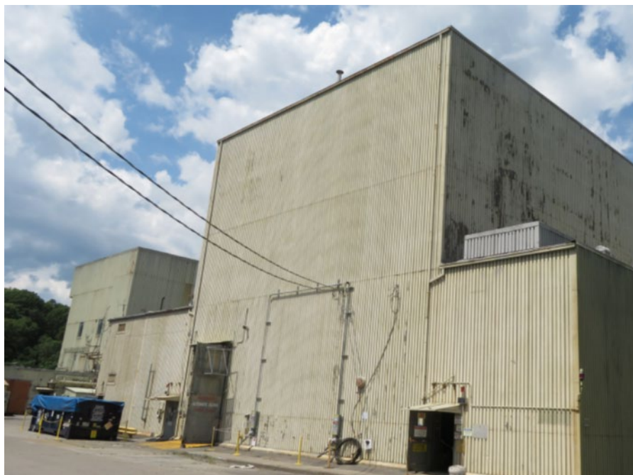
Fig. 6. The west elevation of Building 3042, circa June 2021.
