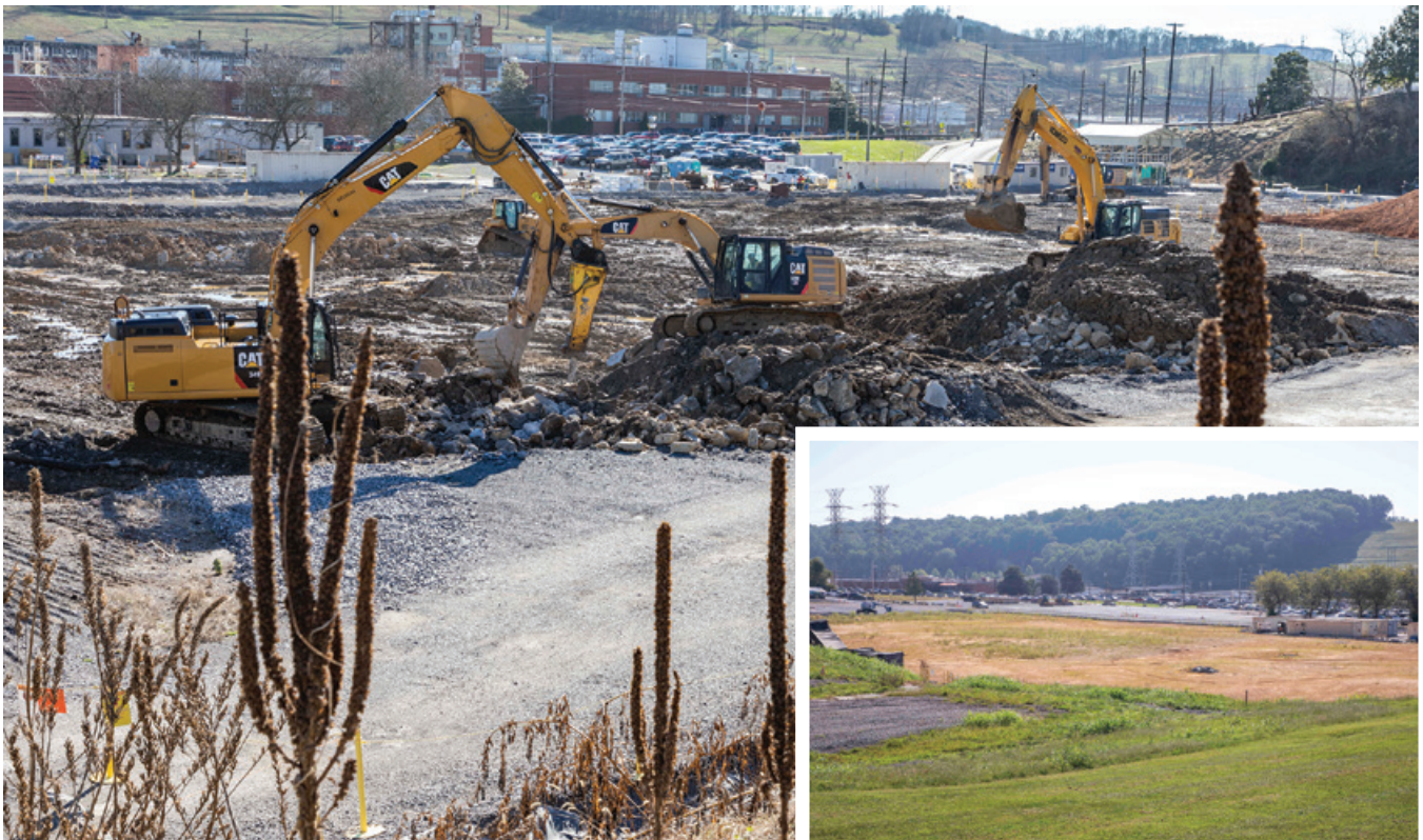
Removal of the Biology Complex slab and completed site (photo inset)
