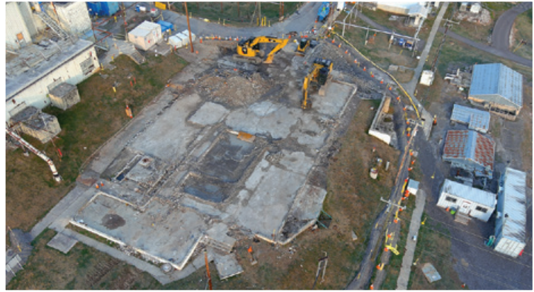
The Bulk Shielding Reactor during demolition (below) and with demolition completed and debris removed from slab (right)
