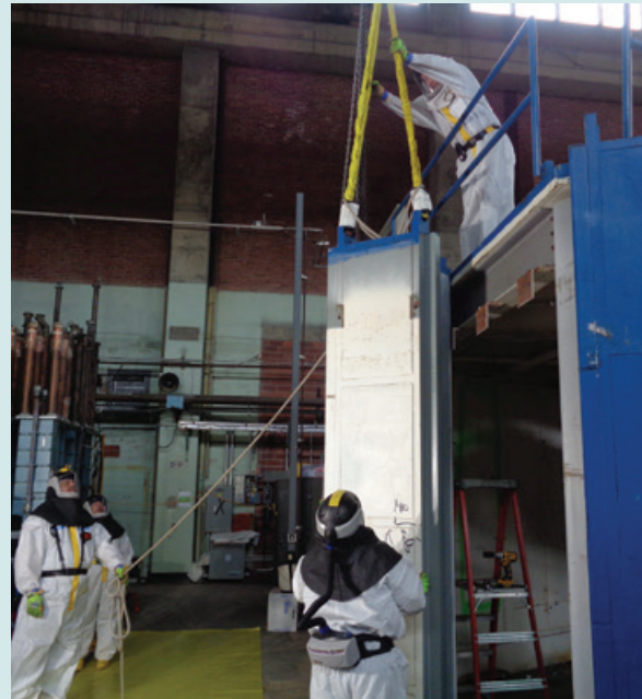
Rigging at Alpha-2
