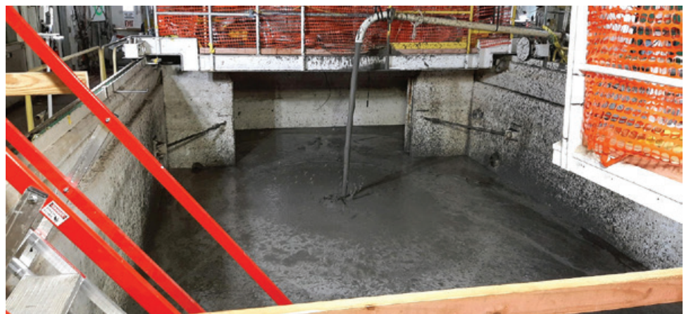
A worker samples the reactor pool wall in the Bulk Shielding Reactor (above left); the reactor pool is filled with a concrete mixture (right); and demolition begins on the facility (above right).
