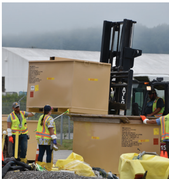
Excavation and packaging of EU-25 waste
