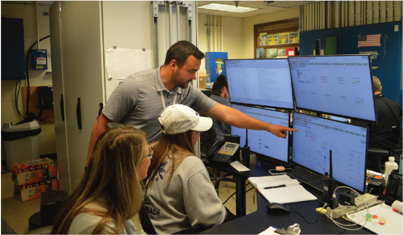
Upgrade of the DCS at LGWO provides 24-hour, real-time monitoring of the entire system.
