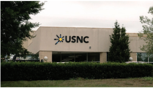
Ultra Safe Nuclear Corporation established a first-of-a-kind pilot fuel manufacturing facility at the Heritage Center to produce its proprietary nuclear fuel.
