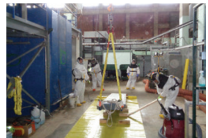
Alpha-2 prep for demolition
