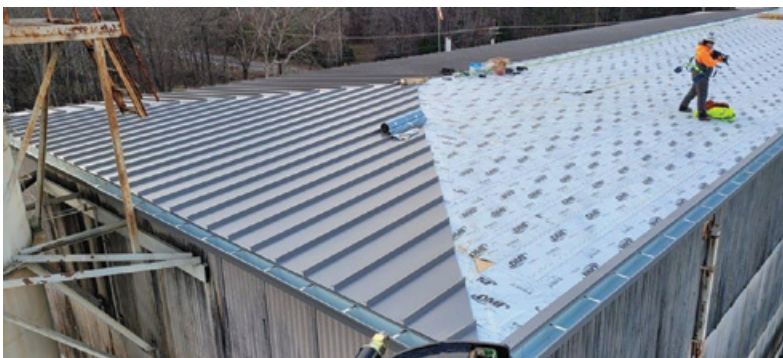
MSRE new roof installation
