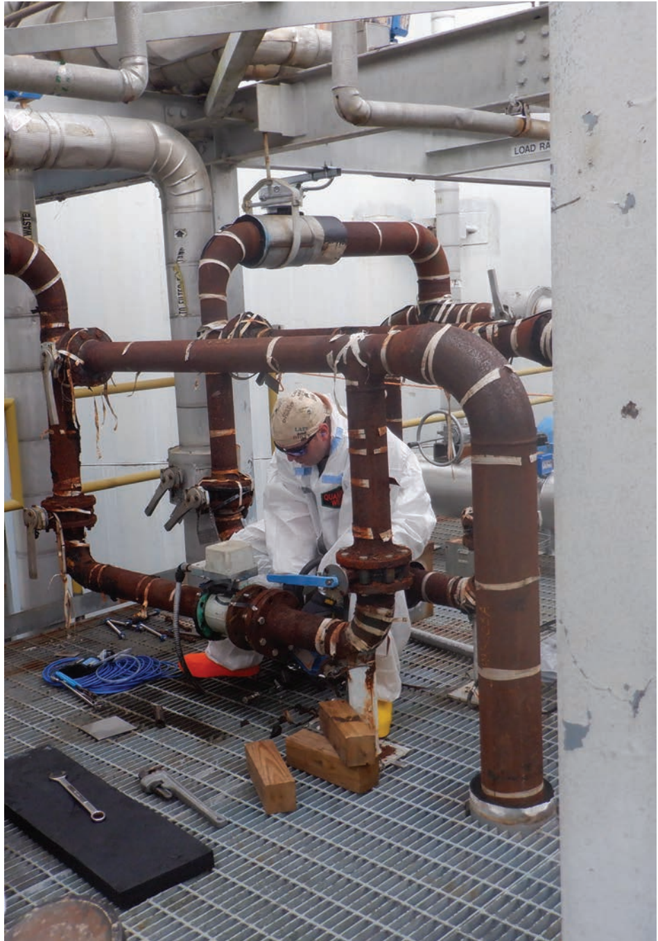
Piping replacement in the 3608 Building
