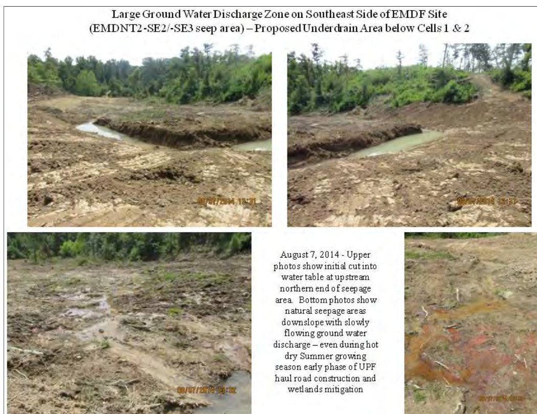
Figure E-64. Early UPF Wetlands Construction of Seep/Groundwater Discharge Area, Southeast Side, Site 5
