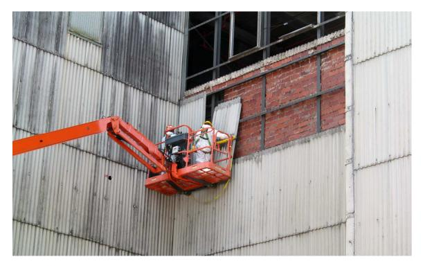
Photo caption (K-25 transite removal.jpg): More than 2,800 transite panels will be removed from the remainder of the K-25 Building.
