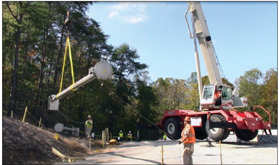
An MSRE salt probe is being positioned for nondestructive assay.
