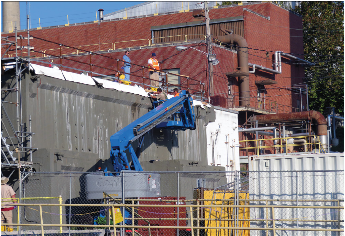
Workers place a fiber membrane on the roof of the 3026-D hot cells to prevent intrusion of rain water into the cells.
