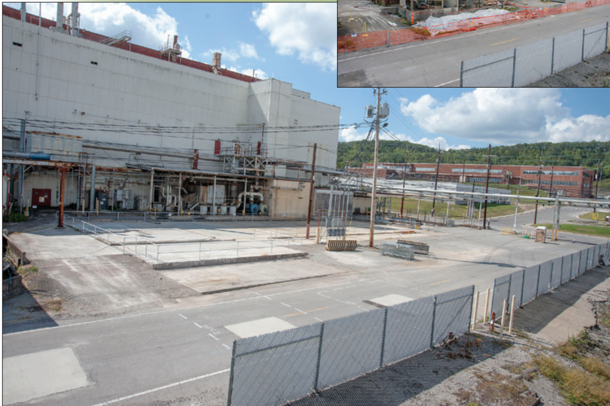
Building 9808 before demolition (right) and after (below).
