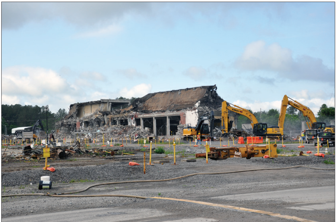
Demolition of Building K-761 Switch House.
