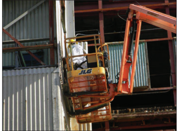
Transite paneling removal.
