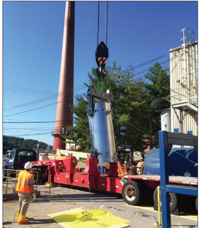
Workers load cask onto transport truck.
