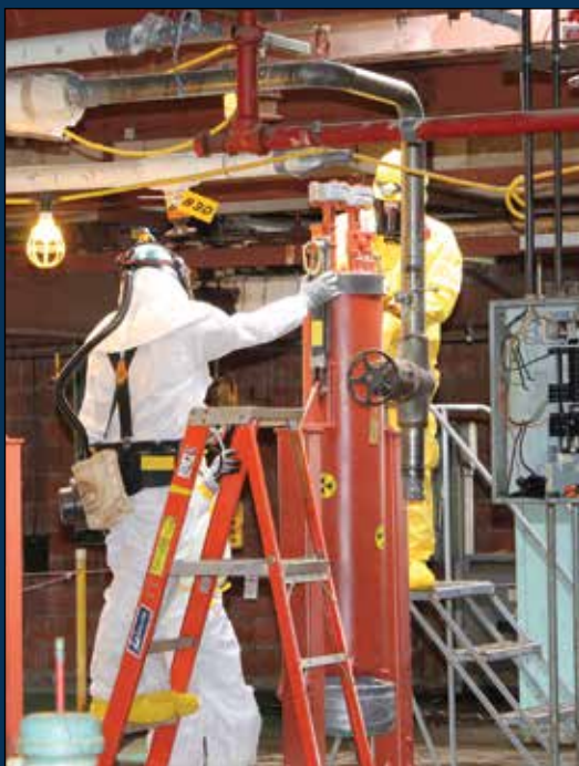
Workers prepare a NaF trap for removal
