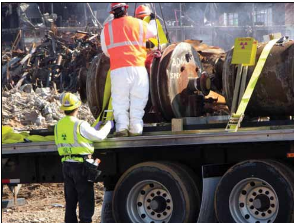
Demolition of the west wing is pictured above. Workers are shown in the photo to the left loading converters removed from the west wing onto a flatbed truck for disposal.
