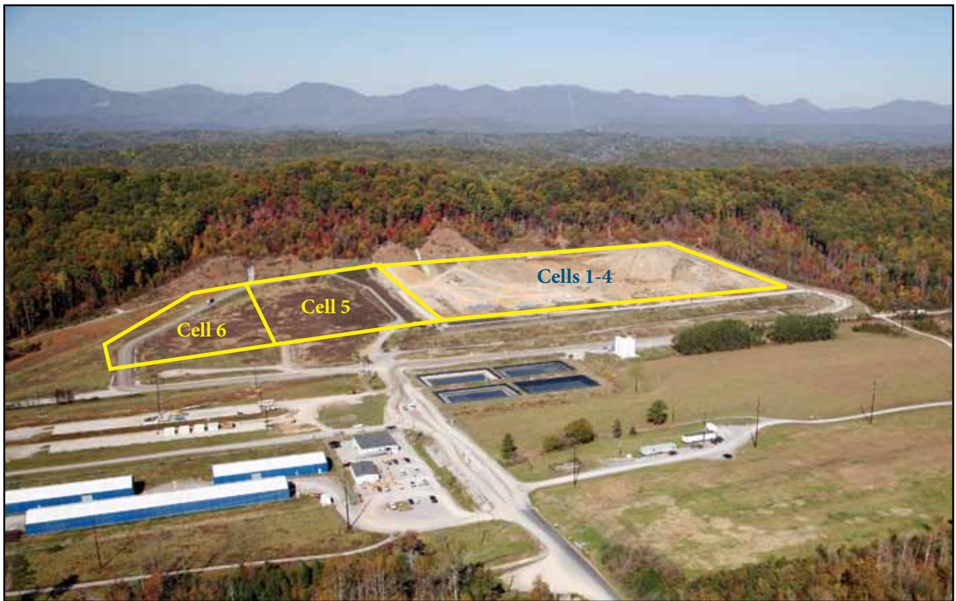
Environmental Management Waste Management Facility
