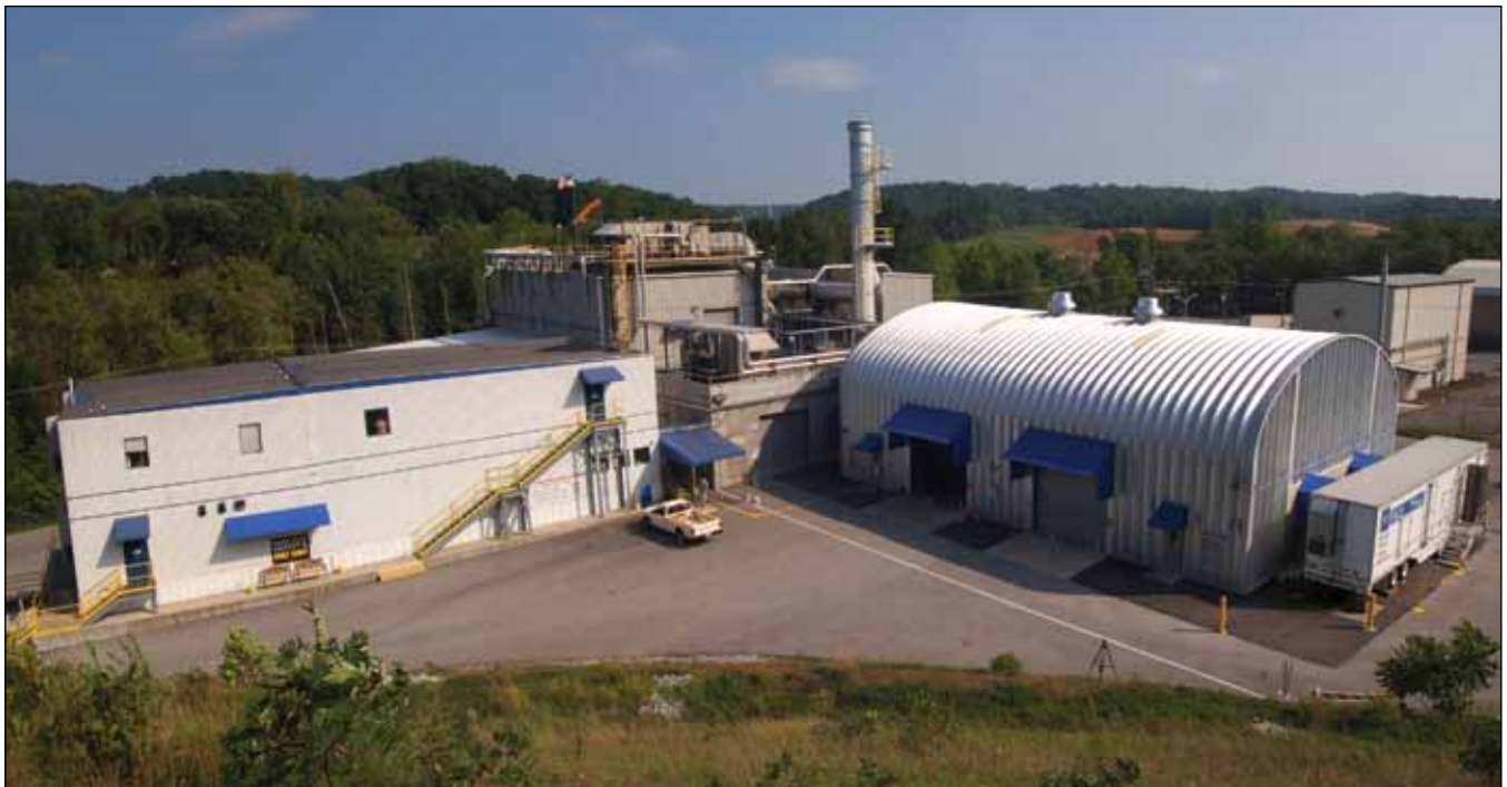
Transuranic Waste Facility
