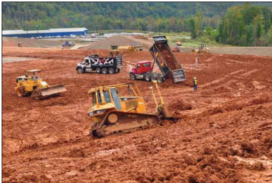
Cell construction at EMWMF
