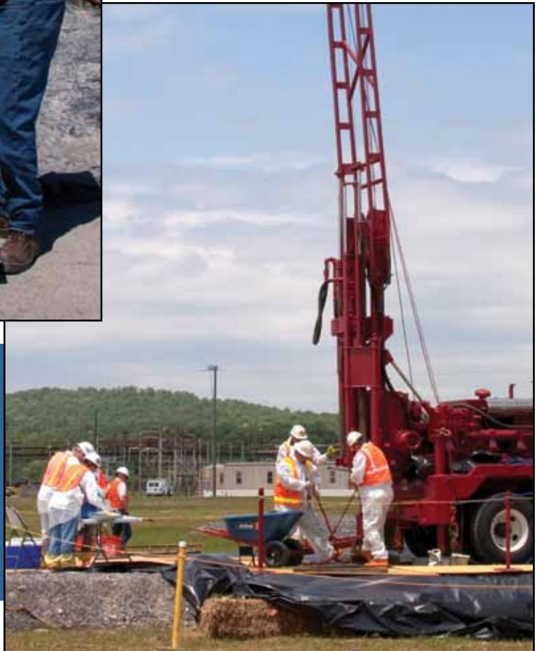
A drill rig is being set up to take core samples.
