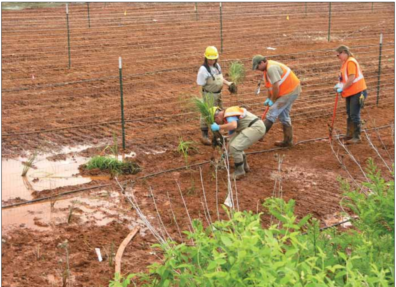
Workers are revegetating an area near an ETPP holding pond that was recontoured in FY 2009.
