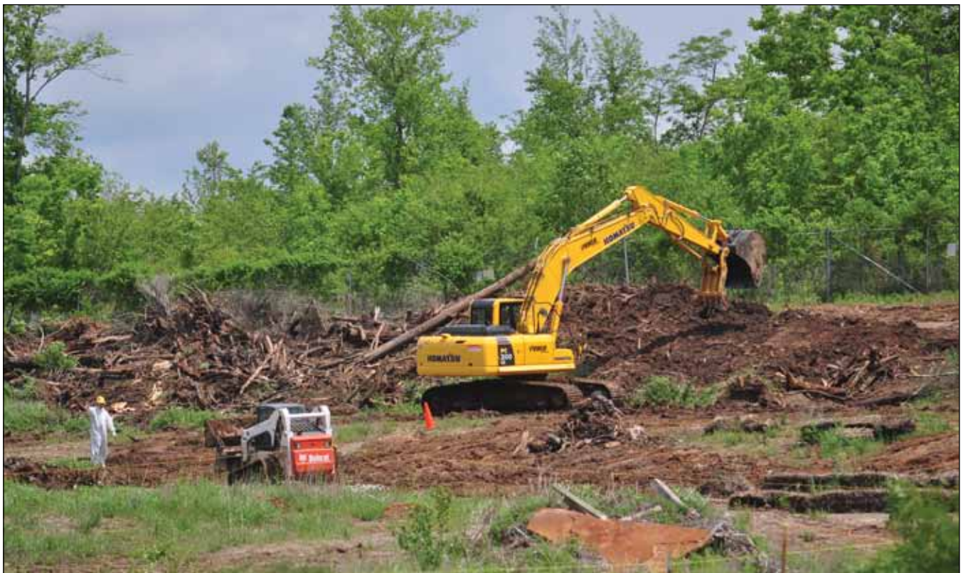
Excavation of contaminated soil at the K-770 area
