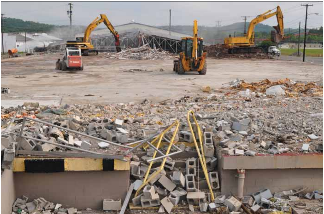
Workers completed demolition of the K-1035 Building, a former maintenance and instrument shop, in the summer of 2009.
