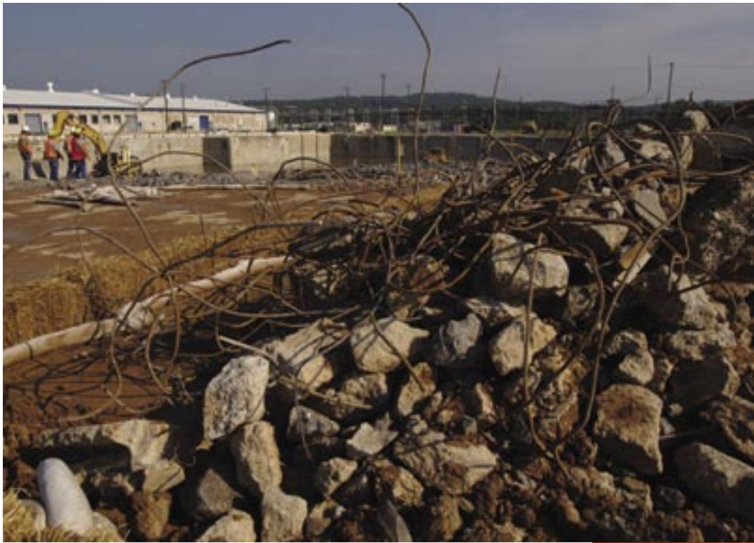
The slab debris, left, provides suitable backfill material for the K-1401 basement. Below, Foreman Becky Phillips and Project Manager Lydia Birk discuss slab demolition at the site.
