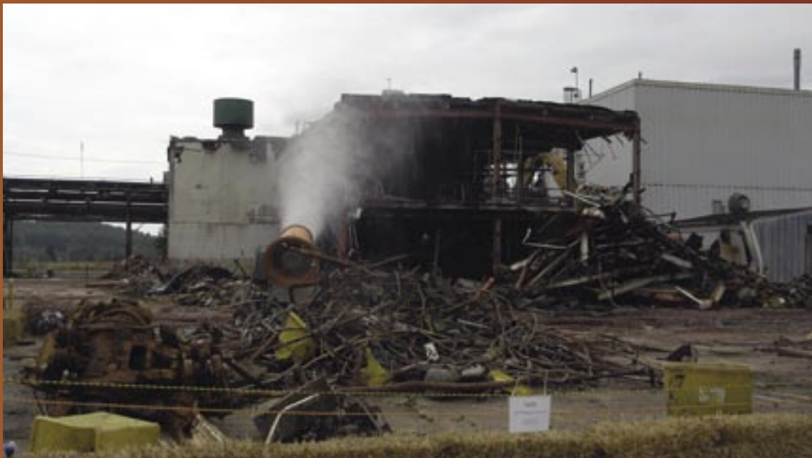
Demolition of K-413, a gaseous diffusion process support building
