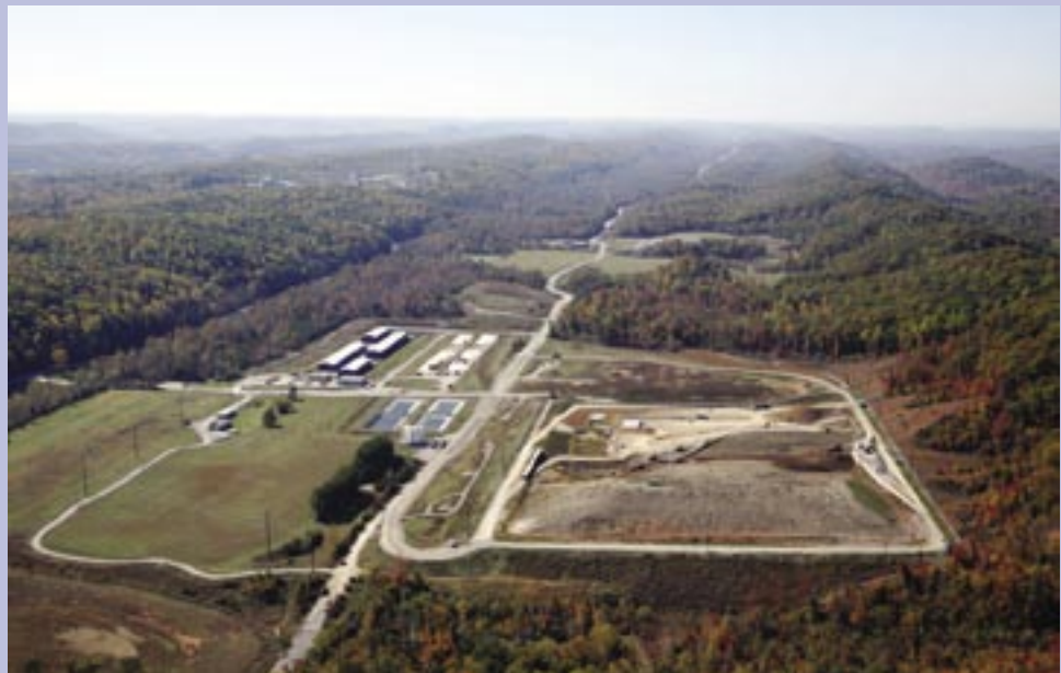
CERCLA Waste Facility, with a view of the haul road winding through the Reservation.
