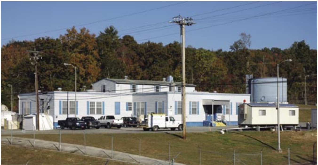
The K-1515 Water Treatment Plant Complex has been transitioned to the City of Oak Ridge.
