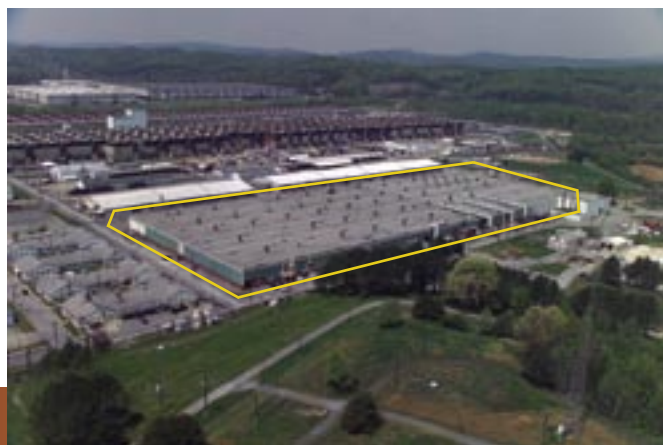
Building K-1401 before demolition
