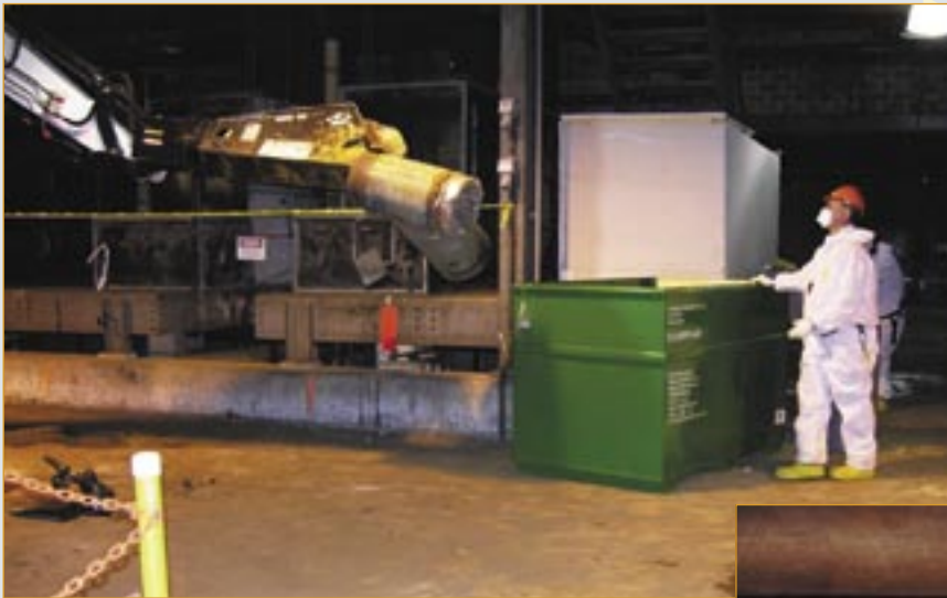
A valve removed from the building process gas system in the K-25 building is being loaded into a box for shipment to the Nevada Test Site.
