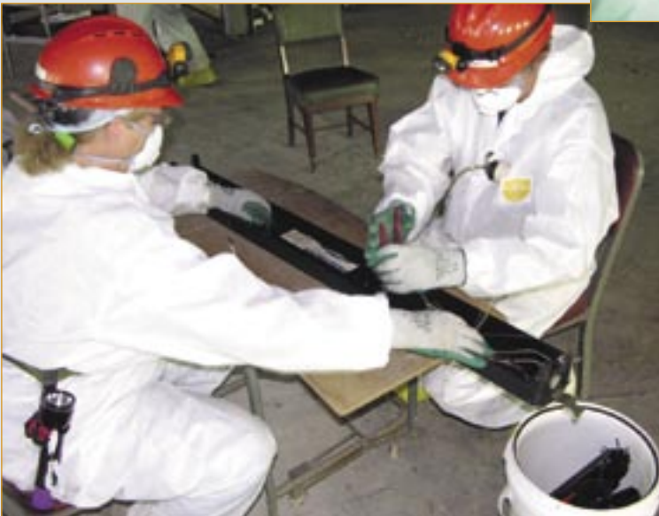
Workers are removing light ballasts for the K-312 section of the K-25 building. About 2,700 light fixtures will need to be removed.
