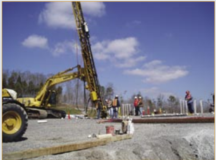
Driving sleeve pipes at Trench 7
