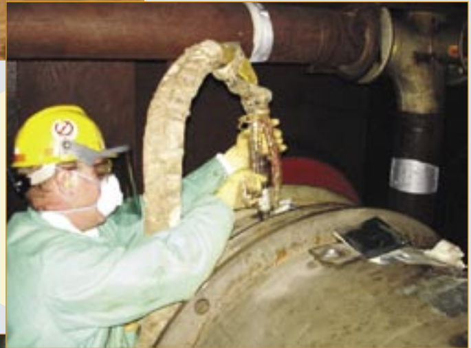
Process equipment is being foamed for contamination control. The foam solidifies contaminants in place.
