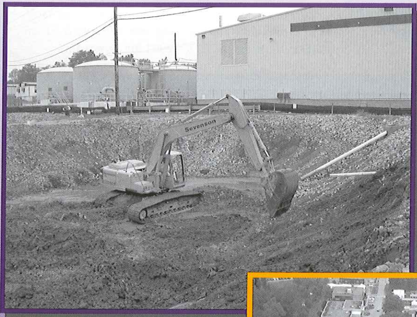
Excavation of contaminated sediment at HFIR pond
