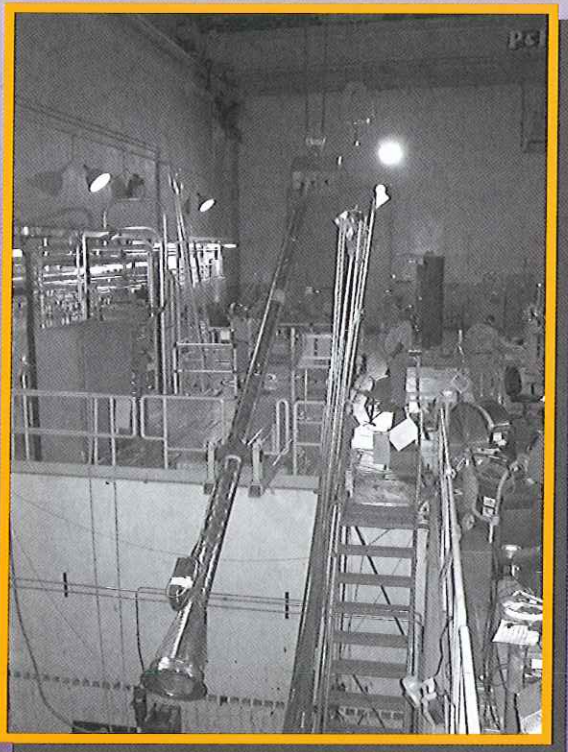
Installation of salt melter probe
