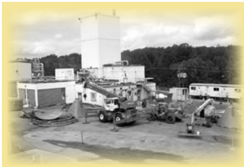
Ongoing demolition of the New Hydrofracture Facility
