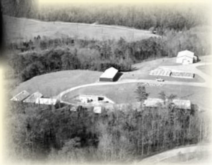
Aerial photograph of SWSA 5 North
