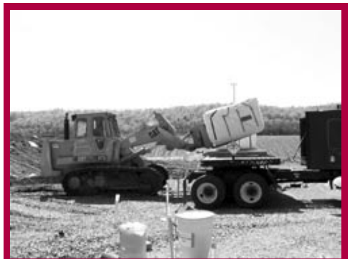
SIOU waste being disposed of at the EMWMF
