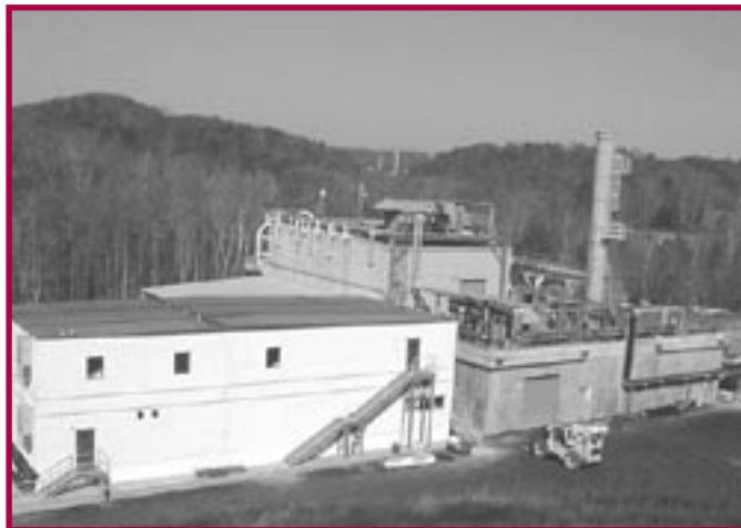
TRU waste processing facility
