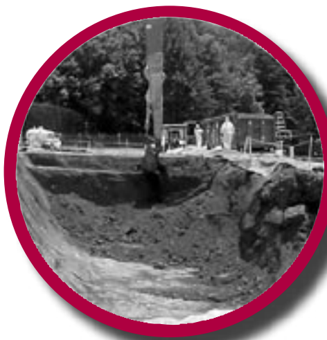
Excavation at K-1070-A
