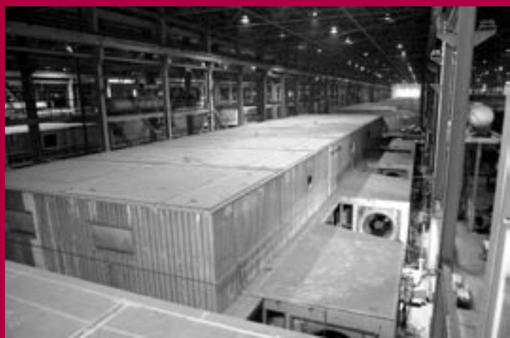
K-33 Cell floor before dismantlement
