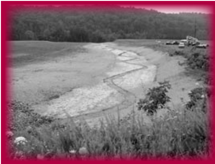
BYBY wastes have been excavated and the site backfilled
