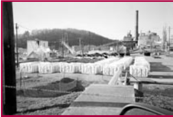
Solidified sediment awaiting final transport to a disposal facility
