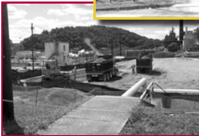
Impoundment 3524 being backfilled
