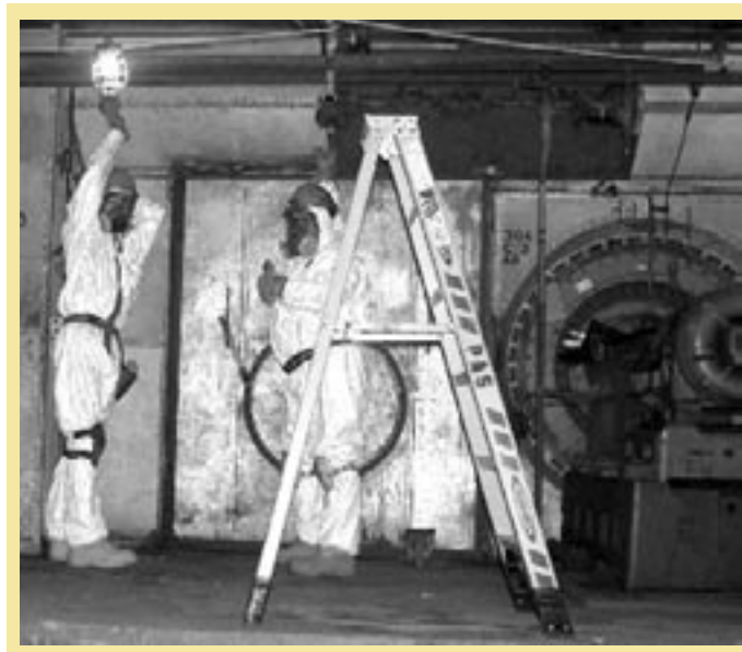
Transite removal from cell enclosure in Building K-25
