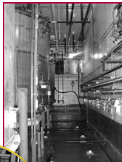
LLW Tank Vault Room
