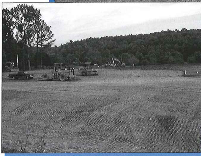
Additional soil and vegetative cover were placed over the Bear Creek Burial Gound D-East site in FY 2002.
