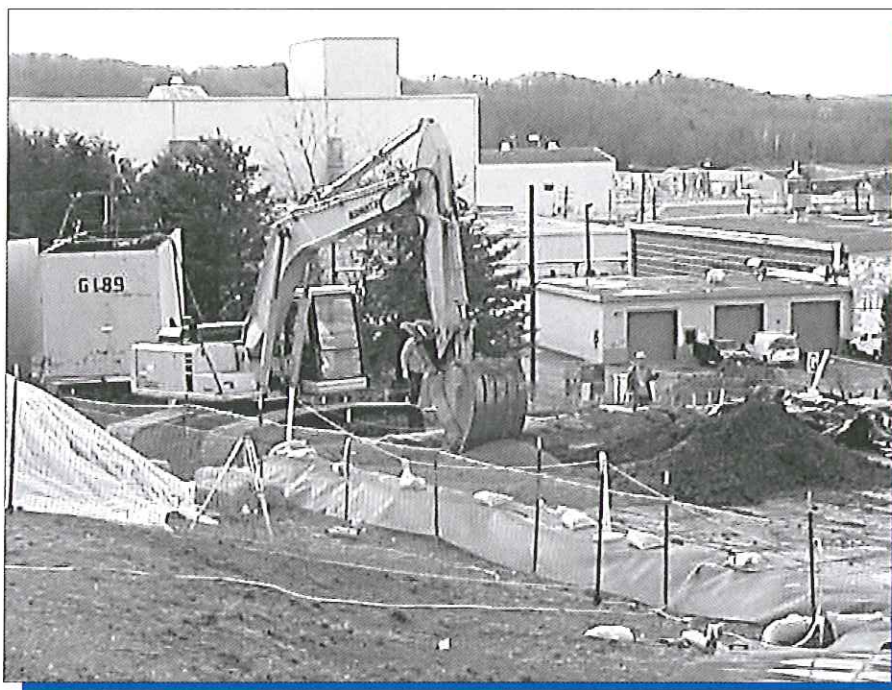
Excavation of buried material at G-Pit was one step in cleaning up the K-1070-C/D burial ground.
