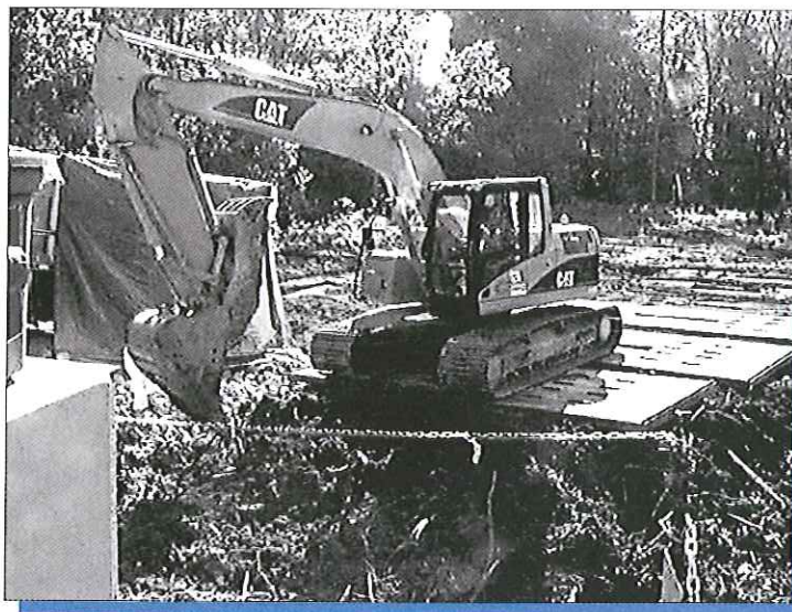
More than 21,000 tons of contaminated soil has been excavated at the Intermediate Holding Pond.
