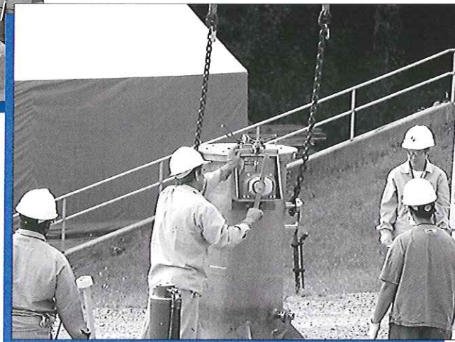
A worker is using a winch to lower a spent nuclear fuel canister into an interim storage position.
