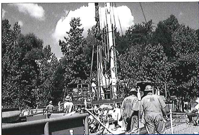
Plugging and abandonment of hydrofracture wells at ORNL continued in FY 2002.
