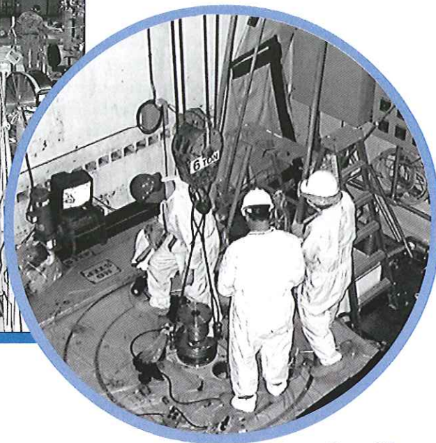
The salt melting probe is being installed over the MSRE Fuel Flush Tank. It assists in the in situ pool melting of the solidified fuel and flush salts.
