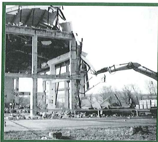
K-1410 during demolition
