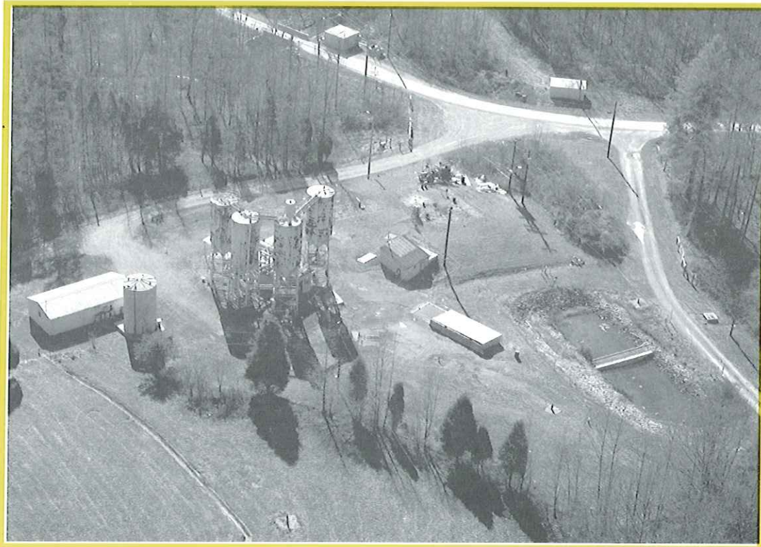
OHF Ponds and Tanks
