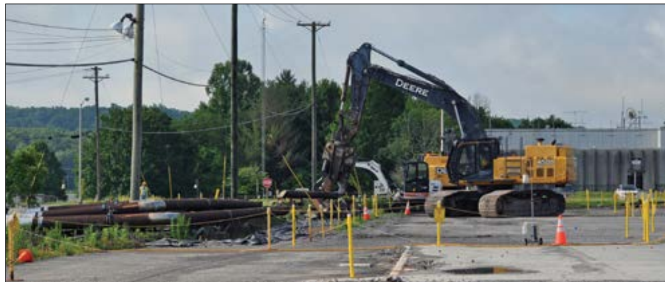
Poplar Creek remediation activities include tie line removal (above) and demolition of the K-832-H Cooling Tower (below)
