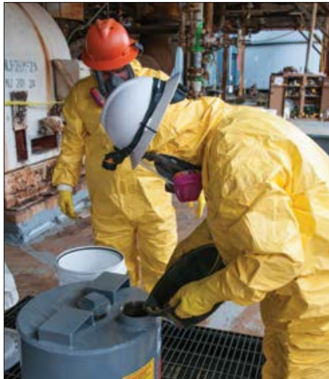
Mercury drained from COLEX equipment is being stored in containers for disposition
