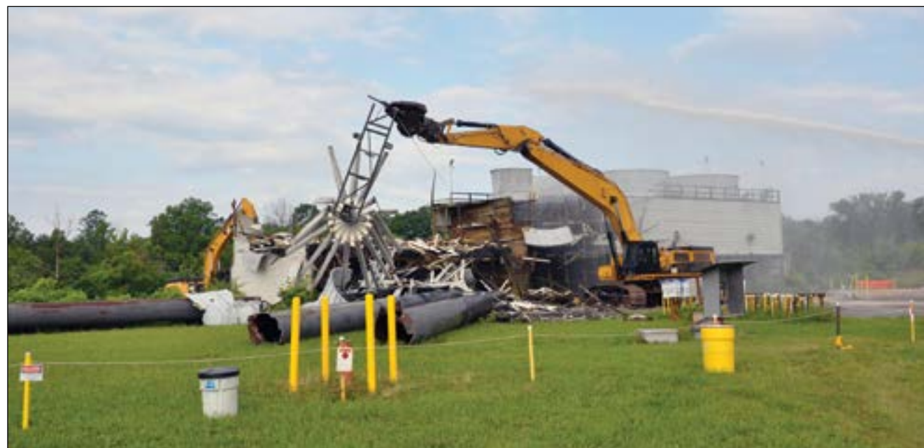
Poplar Creek remediation activities include tie line removal (above) and demolition of the K-832-H Cooling Tower (below)
