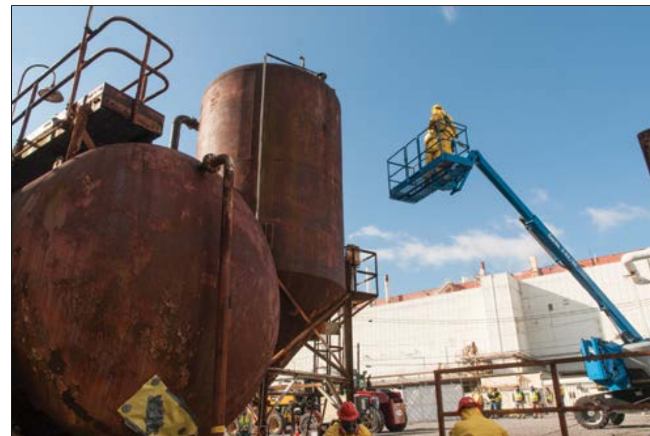
Crews use a man lift to reach a COLEX tank and cut an opening
