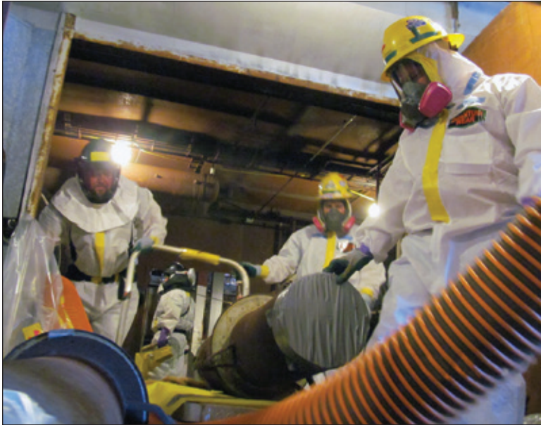
Workers remove process piping in the K-27 Building
