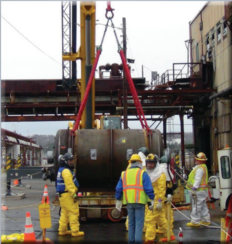
Converter removal from the K-27 Building
