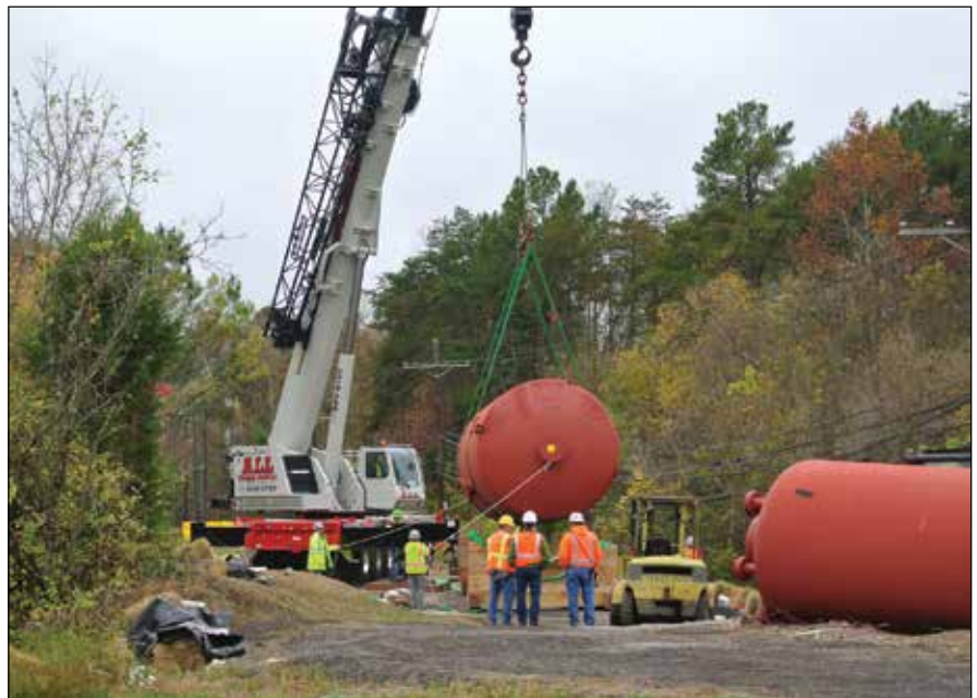
A mercury-contaminated tank is being loaded onto an inspection saddle.
