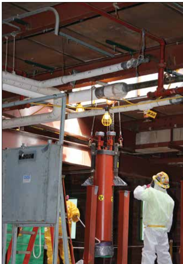
One of the NaF traps that was used in the K-27 Building is being removed.
