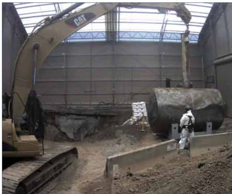
Extraction of Tank W-1A at ORNL
