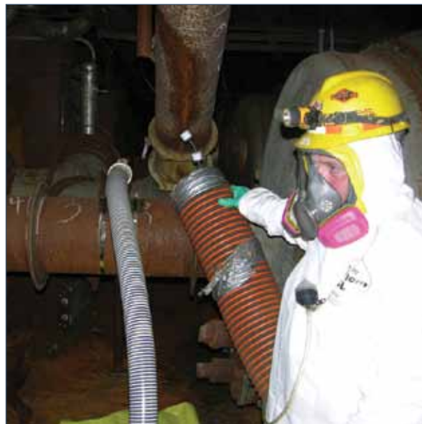
Process equipment in the K-27 Building must go through vent, purge, drain, and inspection steps as part of the pre-demolition process
