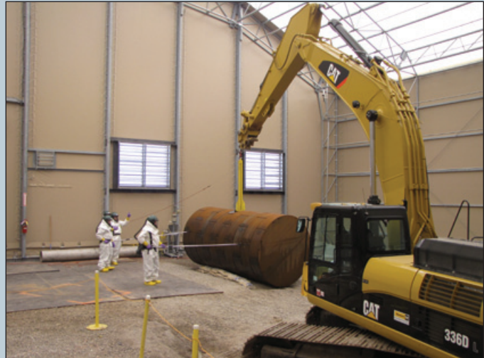
Workers practice tank removal in a specially built structure erected over the excavation site
