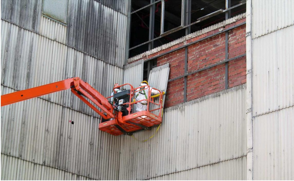
Photo caption (K-25 transite removal.jpg): More than 2,800 transite panels will be removed from the remainder of the K-25 Building.
