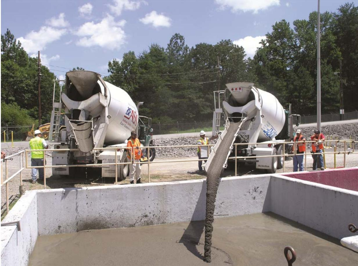
**Cutline for Photo: Workers fill the sumps at TSCAI with grout, as part of closure work.**
