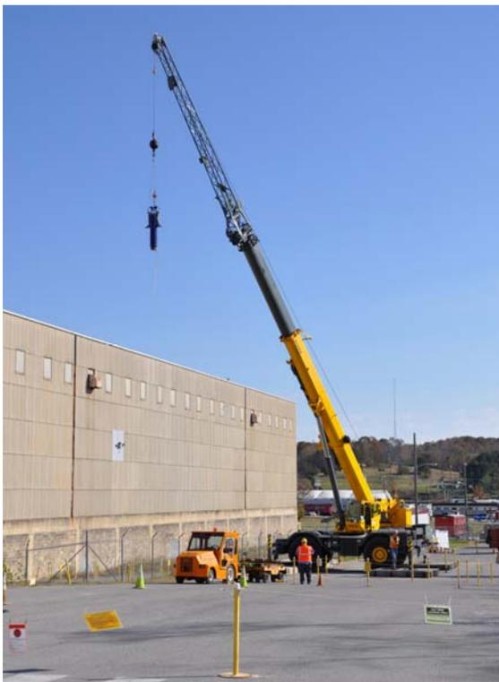
**A crane removes one of five NaF traps from the southernmost portion of K-25’s east wing.**
